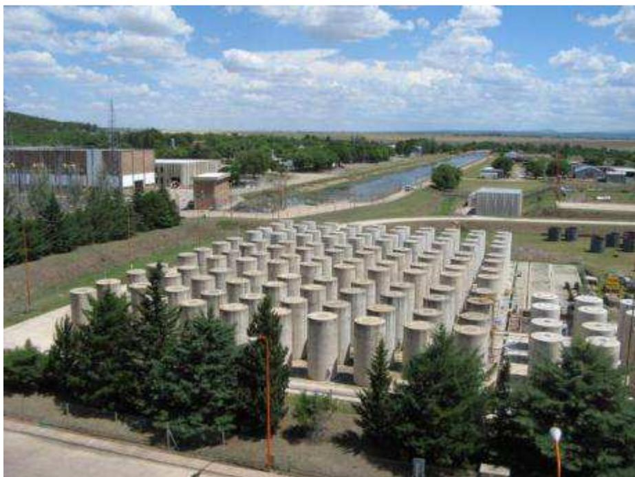
*FIG. 6. Modular array of concrete silos.*
