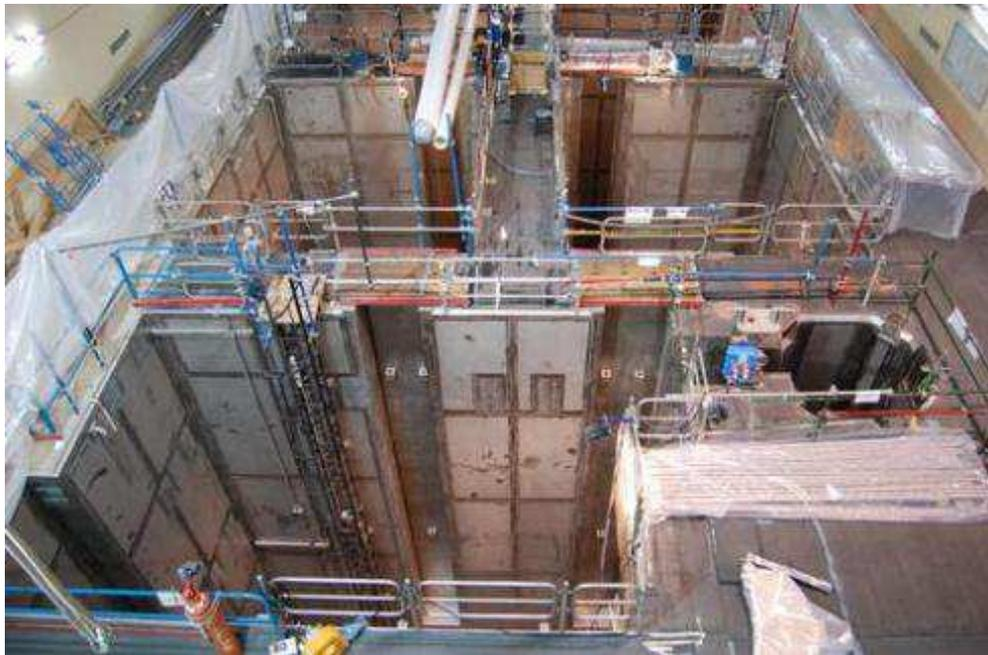
*FIG. 3. The CAN I spent fuel pod (under construction).*
