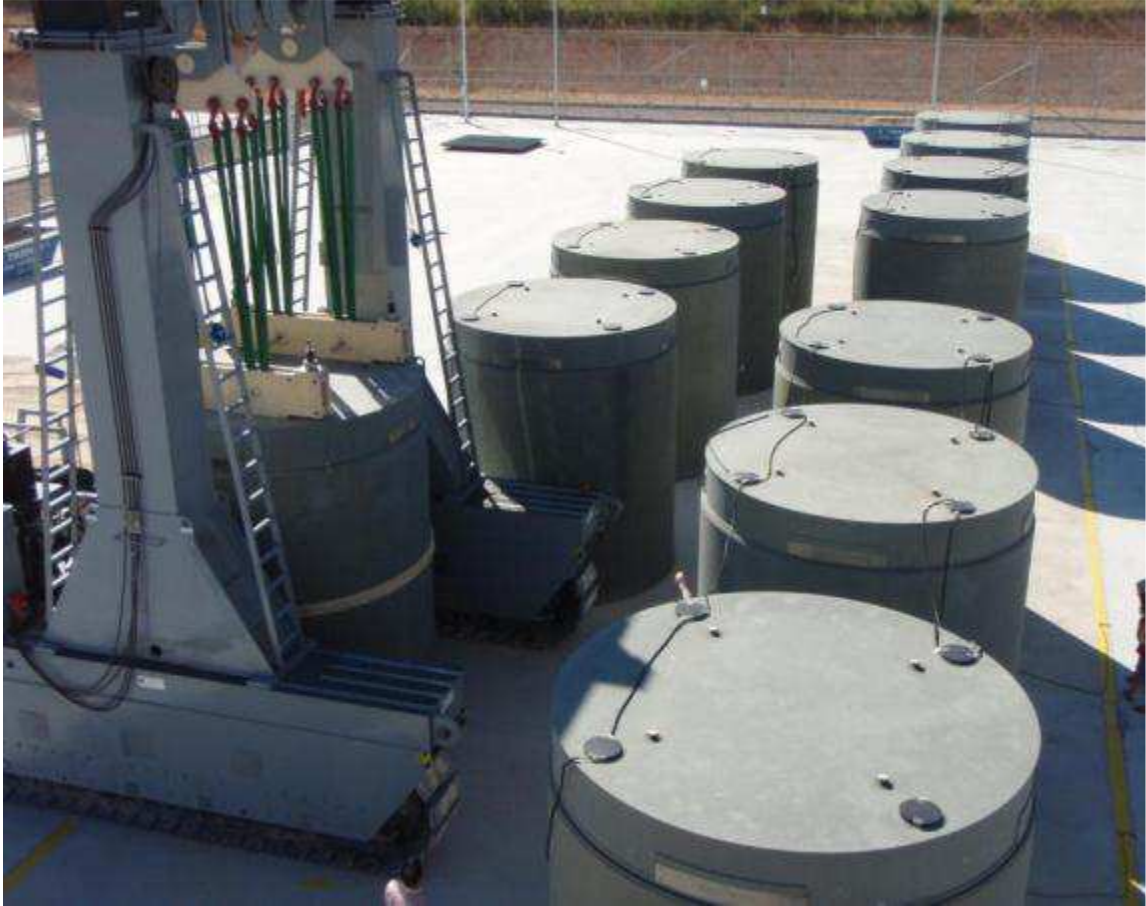
FIG. 1. Trillo NPP dry storage containers.
