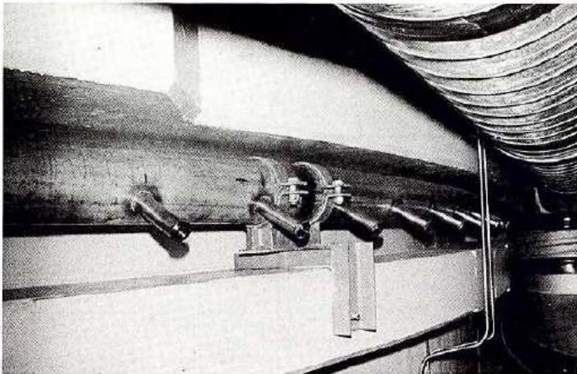
*FIG. 18. System 322 upper containment spray nozzles.*
