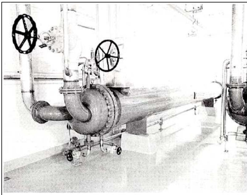
*FIG. 17. System 322 heat-exchanger.*
