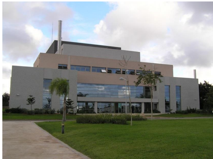
FIG. 1b. CNESTEN TRIGA Mark II Reactor Building and Associated Laboratories.
