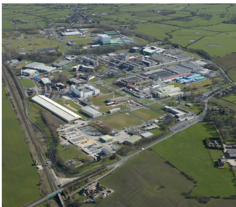
FIG. 1. Springfields fuel fabrication plant.
