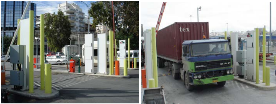
FIG. V-5. Example of a typical vehicle RPM installed at a point of entry.
