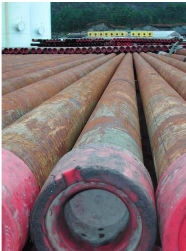
FIG. 15. Oil and gas piping with radium scale — note the end caps used to seal the pipes.
