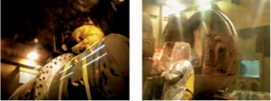
*FIG. 4. Installation of the diamond rope saw in the working caisson and thermal cutting of the low activated part of the KNK reactor rotary lid.*
