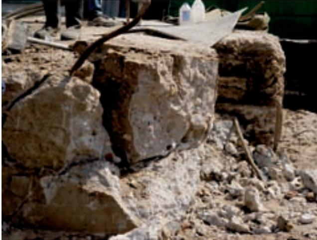
*FIG. 1. Destruction of the in situ concrete cover of repository No. 2 using the electric discharge device.*
