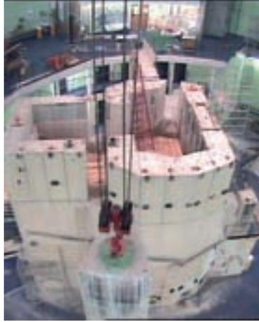
*FIG. 4. Astra reactor, Austria; the biological shield is being removed.*
