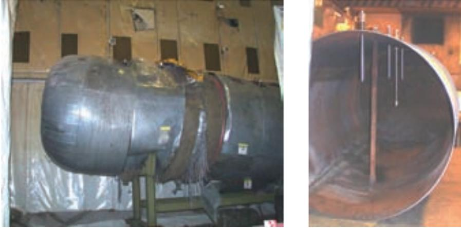
*FIG. 2. Sodium discharge tank during spray moistening for sodium conversion with continuous monitoring of the hydrogen concentration.*
