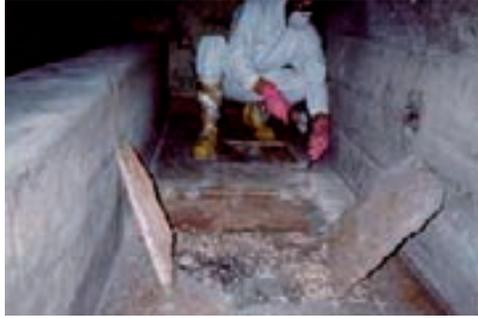
FIG. 2. Removing floor tiles and concrete slabs.
