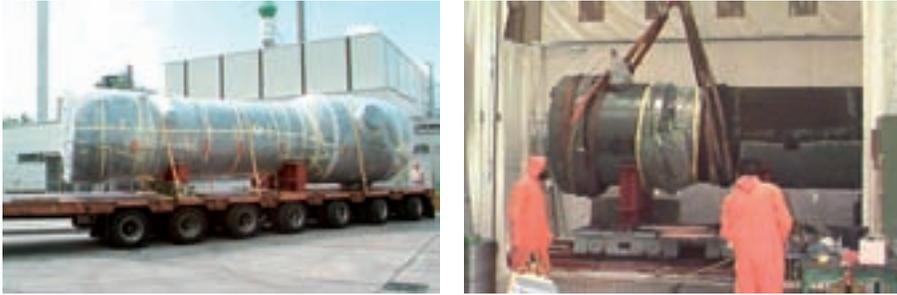
FIG. 1. Transportation and treatment of the MZFR steam generators.
