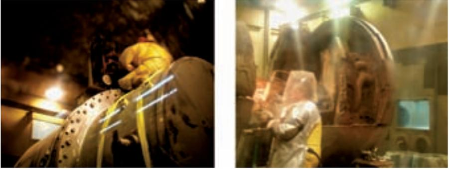
*FIG. 4. Installation of the diamond rope saw in the working caisson and thermal cutting of the low activated part of the KNK reactor rotary lid.*
