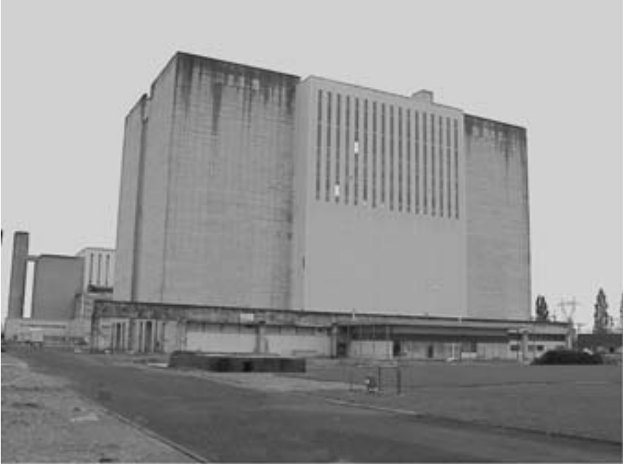
FIG. II-1. The Chinon A2 nuclear power plant.
