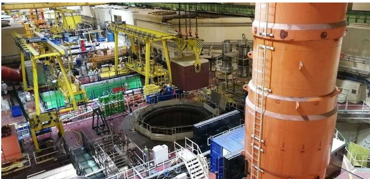
*FIG. 22. Bohunice V1 reactor building during dismantling works (Courtesy of JAVYS)*
