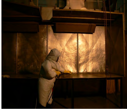
FIG. 8. Example of surface decontamination using steam cleaning. Courtesy of South African Nuclear Energy Corporation.
