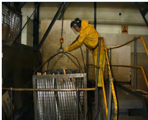
FIG. 7. Removing contamination embedded inside piping. Courtesy of South African Nuclear Energy Corporation.
