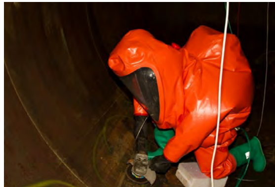
FIG. III–11. Removal of hot spots after water jetting decontamination. Courtesy of Nuclear Research Institute Řež, Czech Republic.
