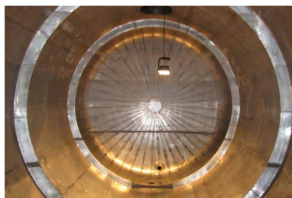
(b) The tank after installation of the stainless steel lining
