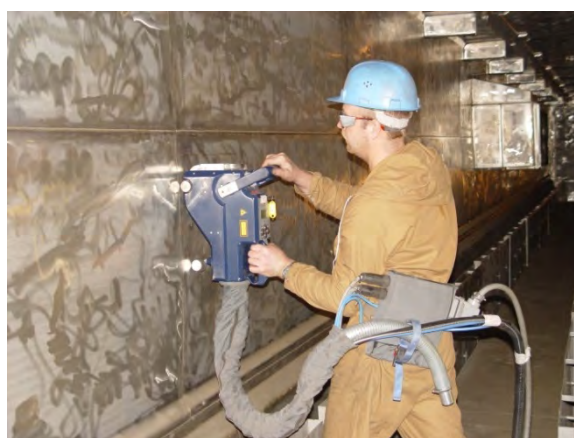
FIG. 4. Laser ablation of metal. Courtesy of Energiewerke Nord GmbH, Germany.
