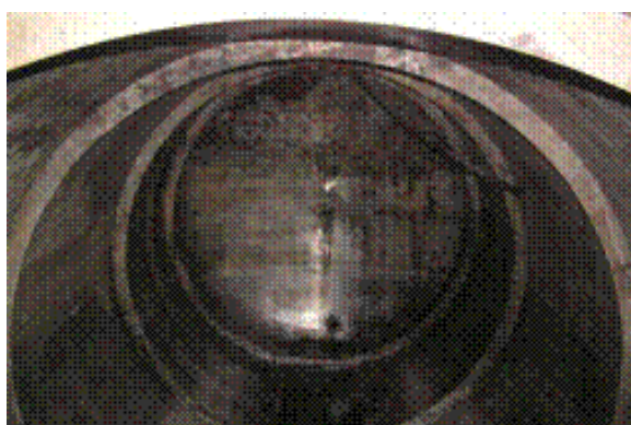
(a) The tank after decontamination before installation of the liner
