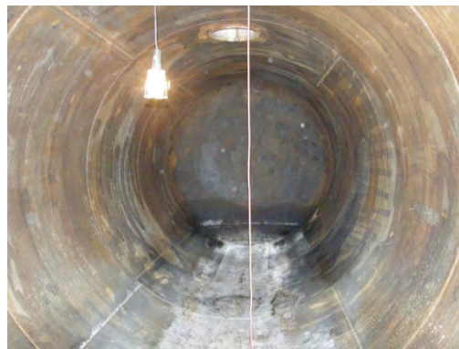
FIG. III–10. Interior of tank B after preliminary decontamination (water jetting decontamination). Courtesy of Nuclear Research Institute Řež, Czech Republic.
