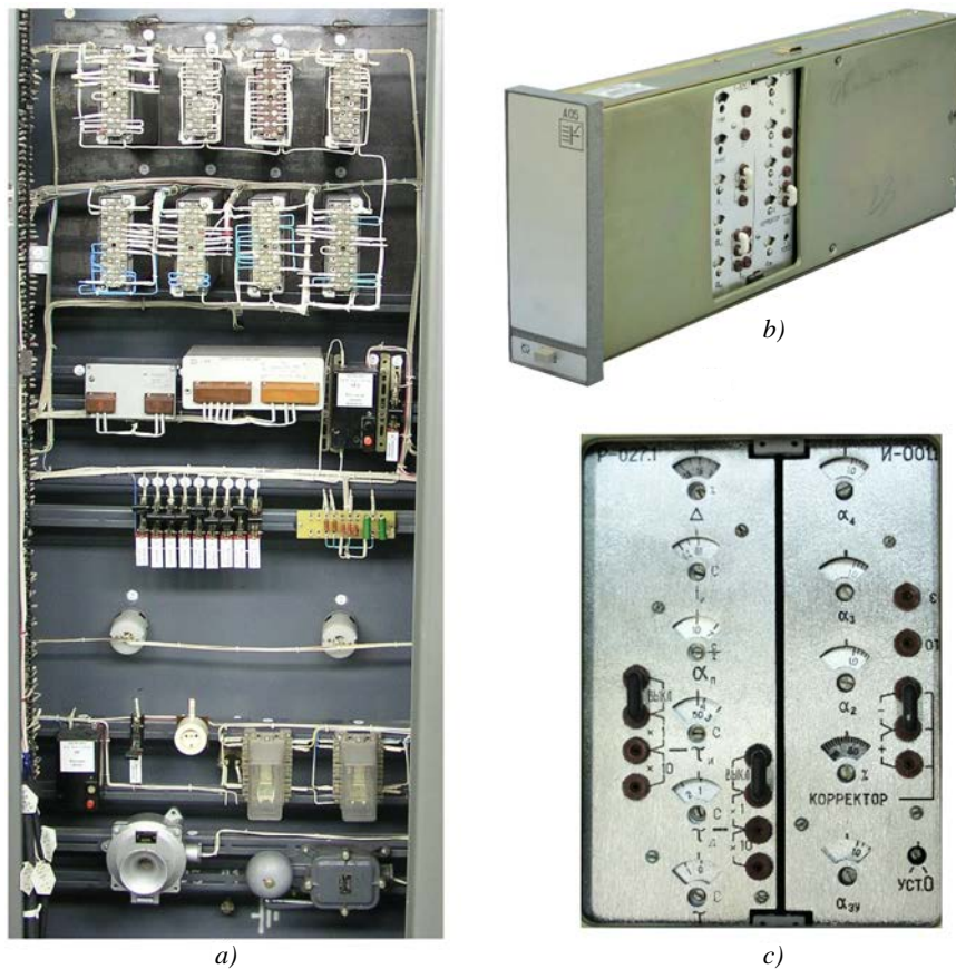
FIG. III-3. External views of the panels and modules of the automatic regulating subsystem before modernization. (a) The regulator panel (rear view); (b) the summation and limiter module; (c) the control module settings panel.
