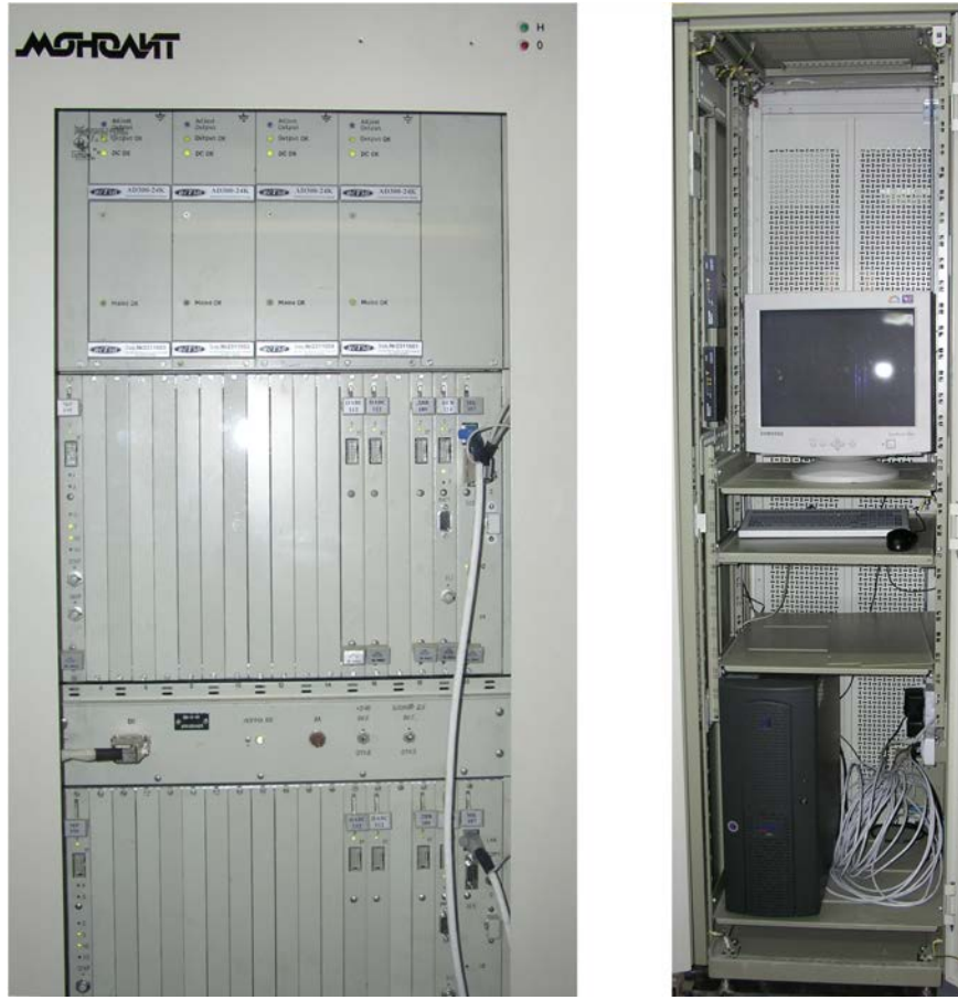
FIG. III-4. External views of the automatic control subsystem of the safety control system after modernization. Left: Regulator cabinet; right: adjusting, diagnostics and historian workstation.
