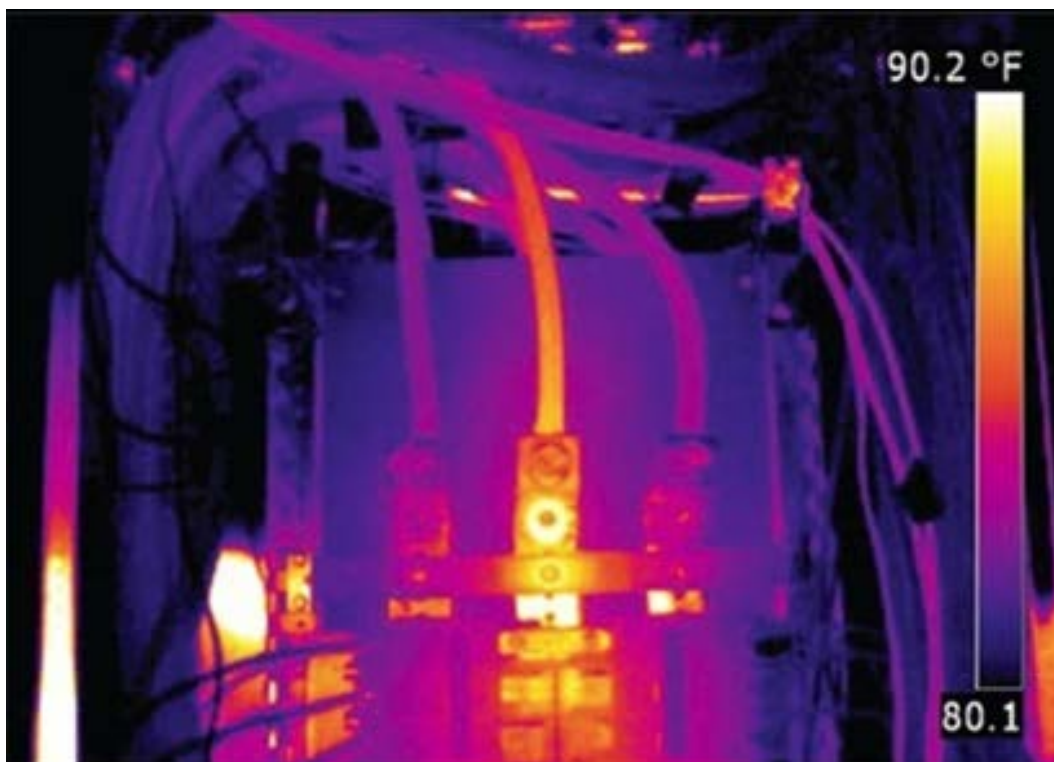
FIG. 9. Heating caused by a degraded equipment cable connector.
