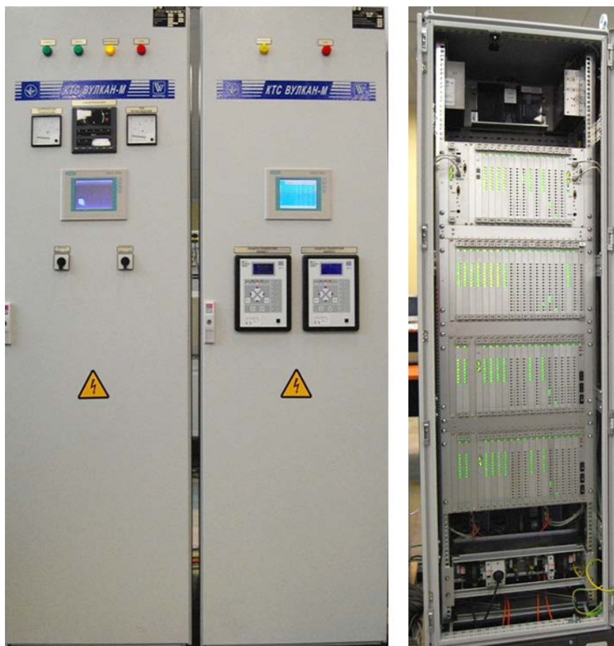
FIG. III-5. General view and internal layout of the cabinet of the safety control system automatic regulation subsystem after the modernization of the SU-1 power unit.
