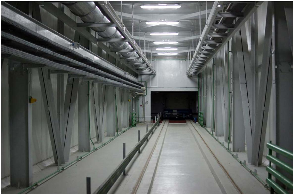
*FIG. 23. Remotely operated dedicated waste container transfer gallery connecting Chornobyl ISRWR to the SRWTP. Courtesy of State Specialized Enterprise Chornobyl NPP.*
