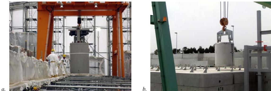
FIG. 39. HICs used for storing slurry and spent adsorbents from treatment of contaminated water at Fukushima: (a) at the ALPS and (b) at the storage area. Courtesy of Tokyo Electric Power Company
