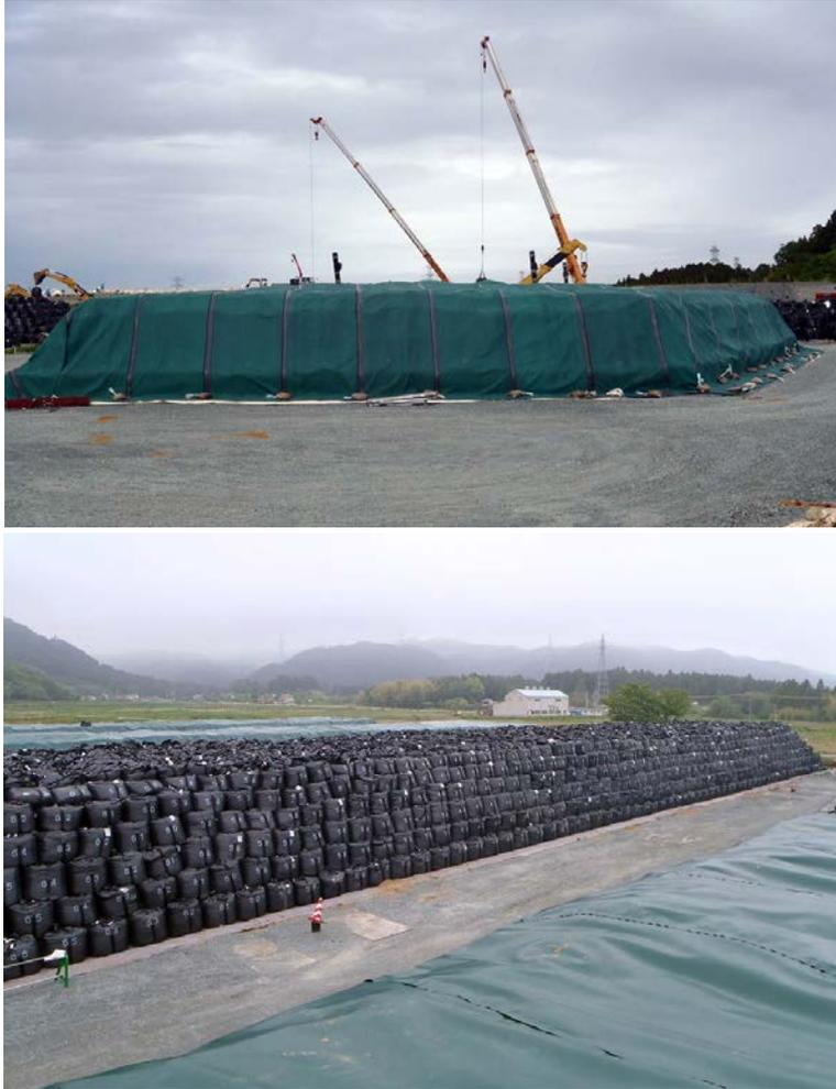
*FIG. 45. Temporary collection sites for contaminated soil and debris at Okuma Town, Fukushima Prefecture. Courtesy of Okuma Town.*
