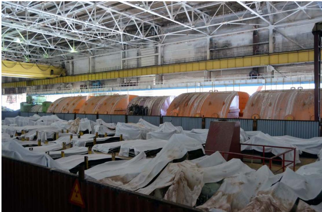
FIG. 6. Temporary (buffer) storage in Chernobyl NPP Unit 3 turbine hall, with fragments of the dismantled ventilation stack from Units 3 and 4. Courtesy of State Special Enterprise Chernobyl NPP.
