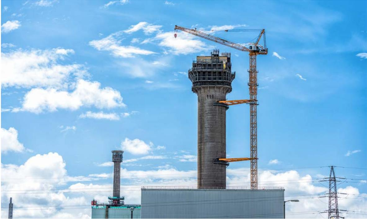
FIG. 20. At Sellafield a 152 m crane was installed to demolish the Windscale Pile 1 chimney. Courtesy of the Nuclear Decommissioning Authority.
