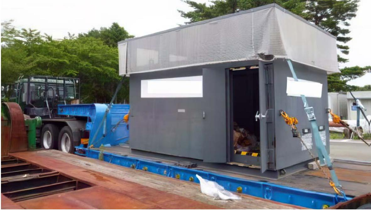
FIG. 30. Mobile treatment system for contaminated water in Fukushima main trench. Courtesy of Tokyo Electric Power Company Holdings.
