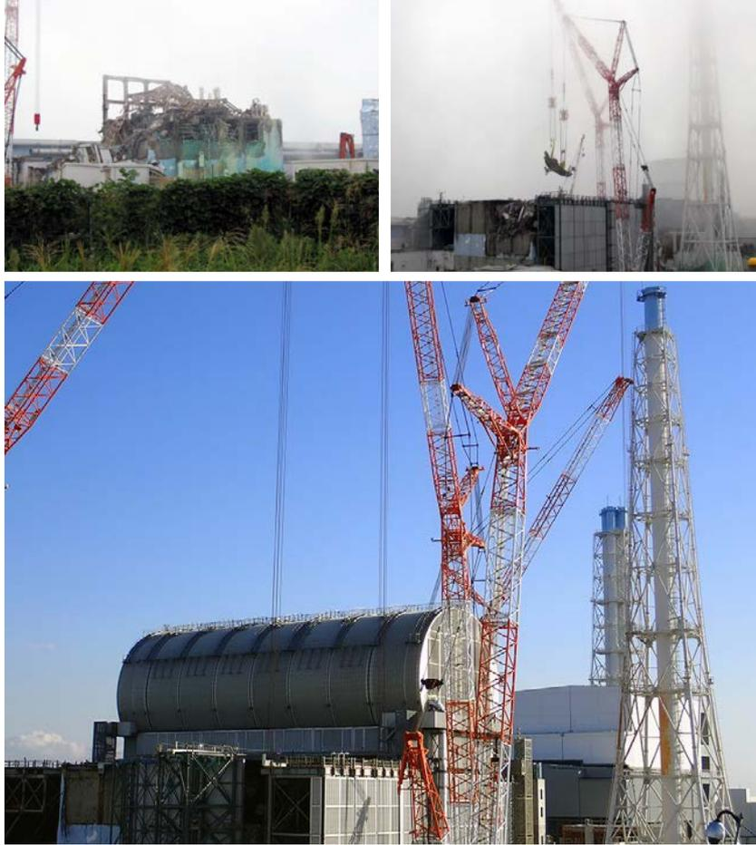
*FIG. 18. Rubble removal and stabilization using cranes at Fukushima Daiichi Unit 3: after the accident — 2011 (top left); during rubble removal — 2015 (top right); current stabilized situation — 2020 (bottom). Upper two photographs courtesy of Tokyo Electric Power Company Holdings.*
