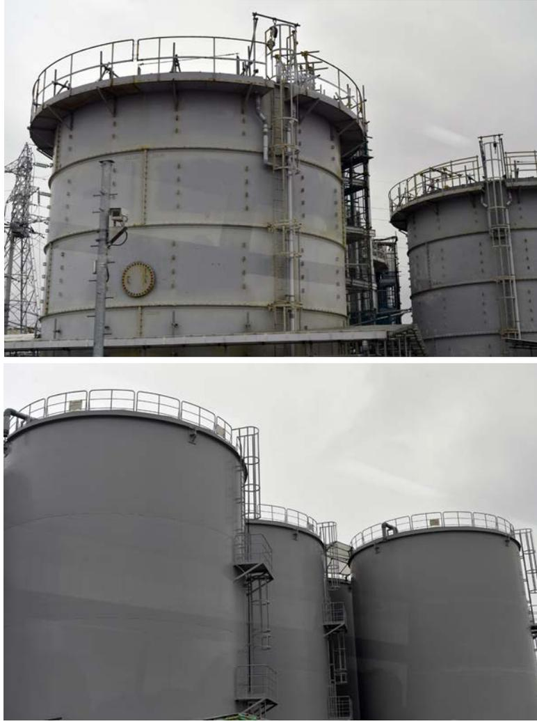
FIG. 47. Bulk contaminated water storage tanks at Fukushima: flanged (top) and welded (bottom). Courtesy of Tokyo Electric Power Company Holdings.
