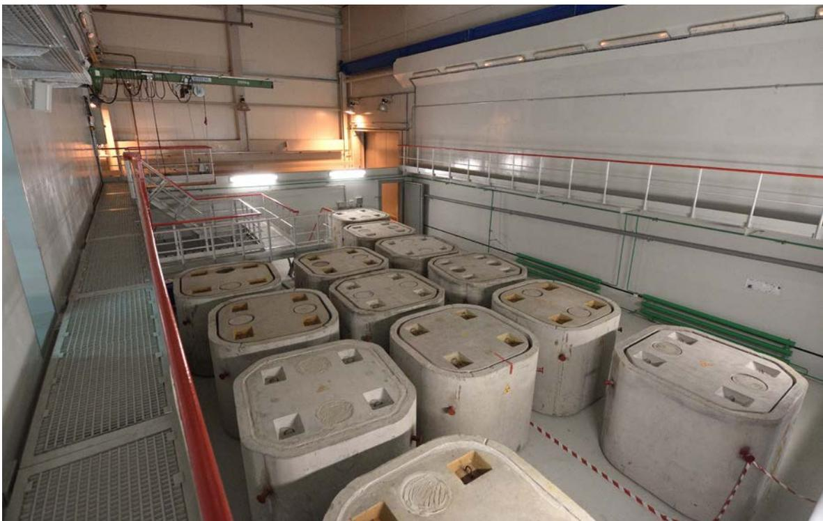
*FIG. 50. Temporary storage facility for solid wastes at the Industrial Complex for Solid Radwaste Management (ICSRM), showing KZ-3 type containers for storage of reprocessed solid low–medium short lived wastes. Courtesy of State Specialized Enterprise Chernobyl NPP.*
