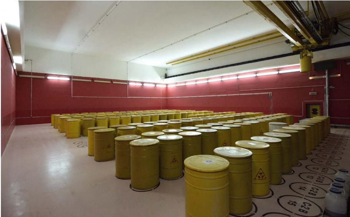
*FIG. 49. Storage hall for treated liquid at Chernobyl Liquid Radwaste Treatment Plant. Courtesy of State Specialized Enterprise Chernobyl NPP.*
