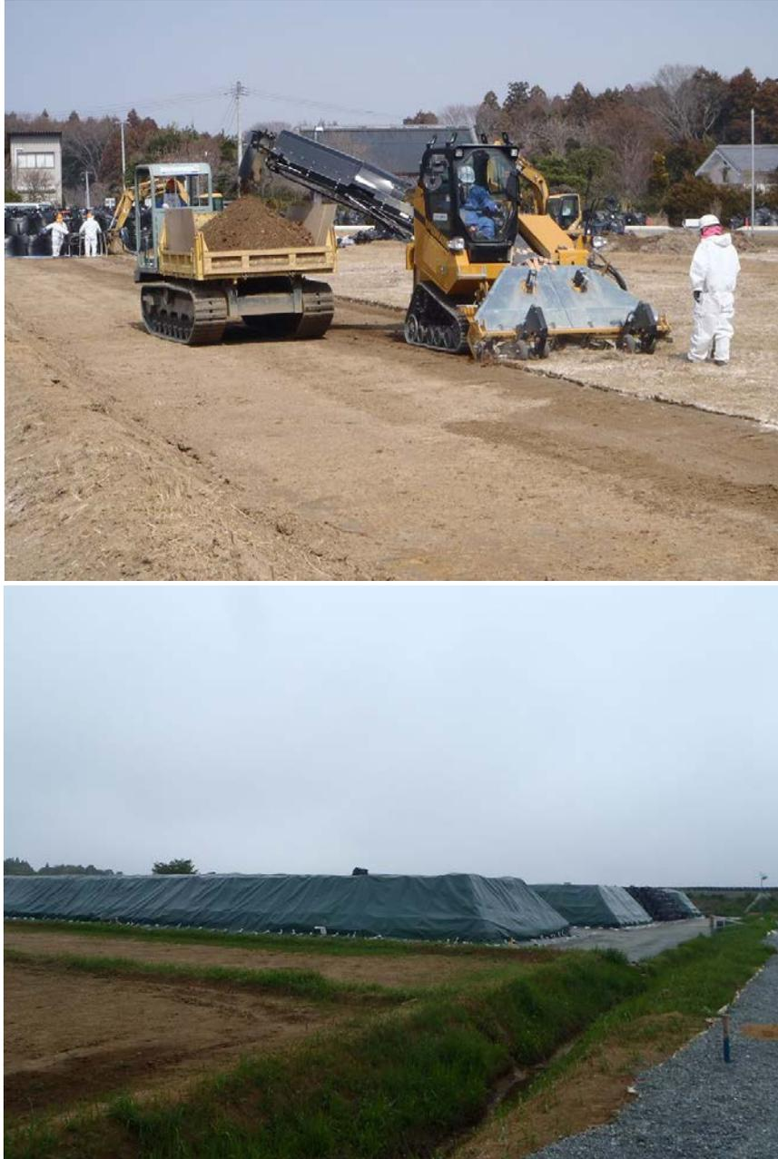
*FIG. 60. Decontamination and collection of soil in an agricultural area (left) and a temporary soil storage facility (right). Courtesy of Okuma Town.*
