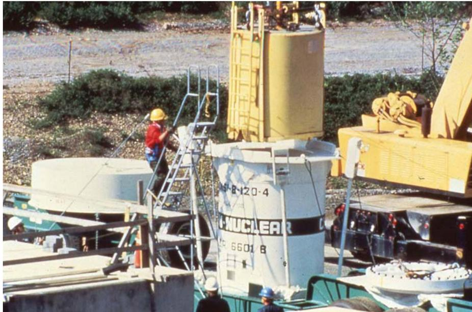
FIG. 42. The CNS 14-190 cask being inspected at TMI. Courtesy of Idaho National Laboratory [25].
