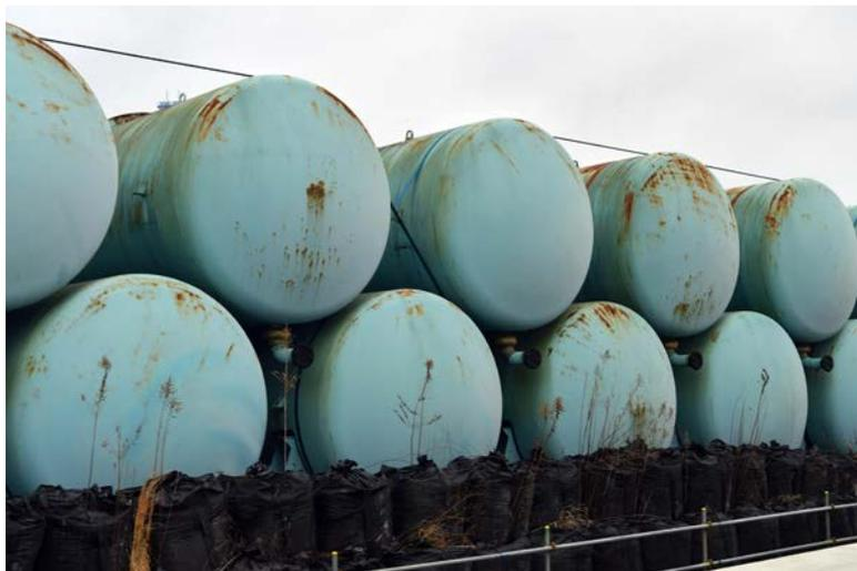
*FIG. 46. Storage tanks for contaminated water at the Fukushima Daiichi NPP.*
