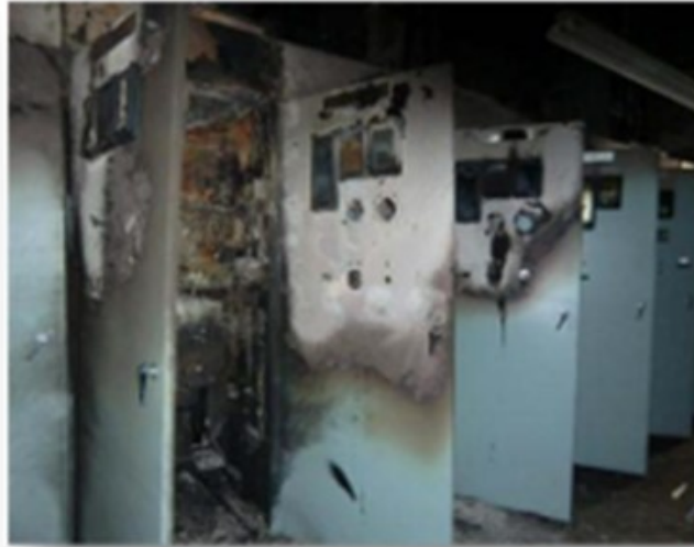
FIG 1. Damage to metal-clad switchgears caused by the Onagawa HEAF event [1]
