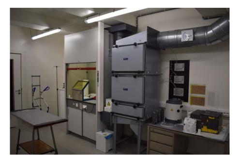
FIG. 23. A 'hot lab' in a veterinary nuclear medicine facility. Manipulation of radioactive material is performed under a fume hood. L-block shielding is present. Note the filter system for trapping airborne radioactive material to the right side of the fume hood. Use of a filter system is mandatory in using volatile radionuclides such as radioiodine. (Courtesy of the Department of Medical Imaging and Small Animal Orthopaedics, Faculty of Veterinary Medicine, Ghent University.)
