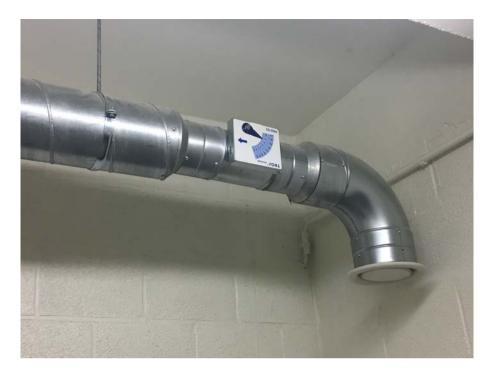
FIG. 19. Piping of the ventilation system to maintain negative pressure in order to reduce contamination and internal exposure of workers when working with aerosols or volatile radionuclides. (Courtesy of the Department of Medical Imaging and Small Animal Orthopaedics, Faculty of Veterinary Medicine, Ghent University.)
