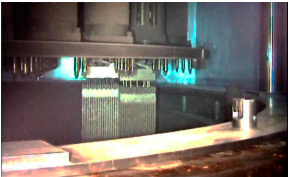
FIG. 29. Two FAs stuck under an upper core plate in a French plant in 2008. Figure courtesy of Électricité de France.
