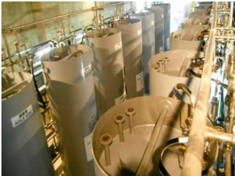
FIG. 24. SARRY vessels in the operating facilities. (Courtesy of TEPCO, Japan.)
