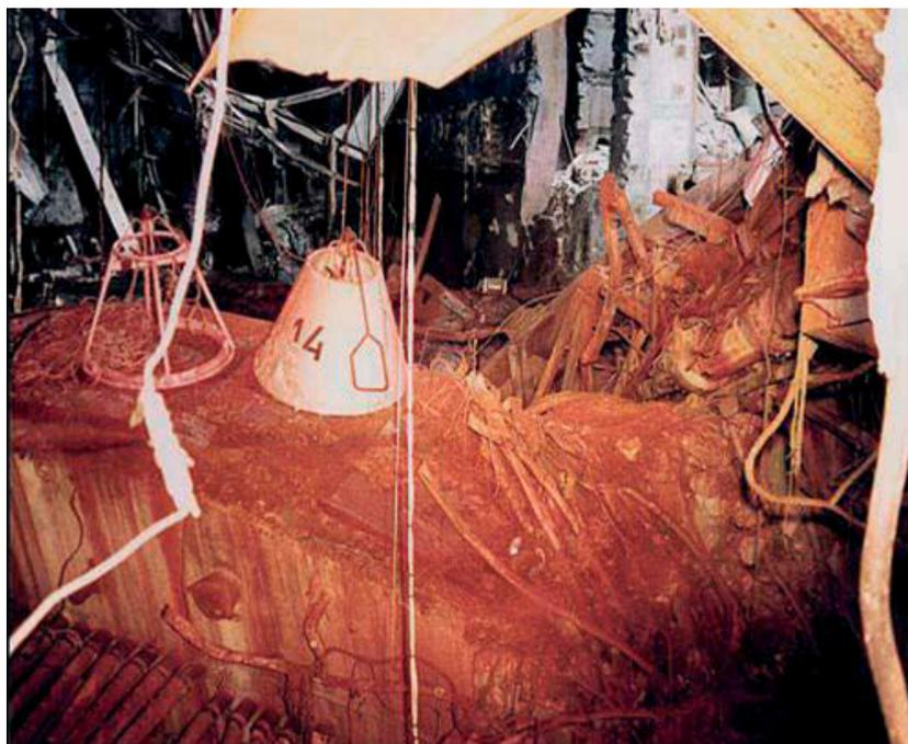
*FIG. 38. The buoy system on the edge of the Elena structure. (Courtesy of Chernobyl NPP, Ukraine.)*
