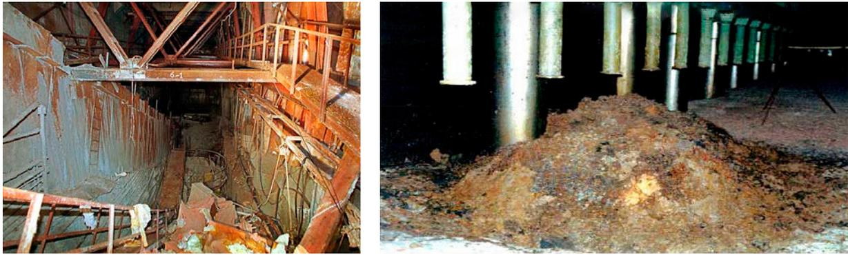
FIG. 26. Debris and material within Unit 4. (Courtesy of Chernobyl NPP, Ukraine.)
