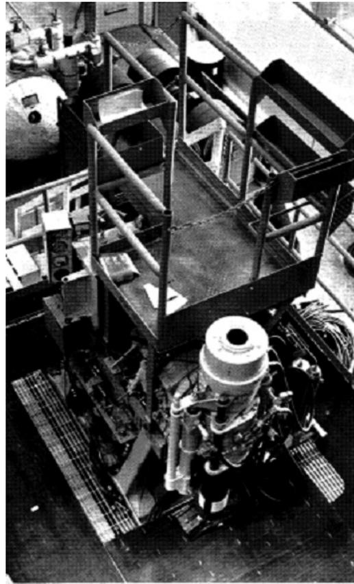
FIG. 42. TMI-2 core drilling machine. (Adapted from Ref. [7].)
