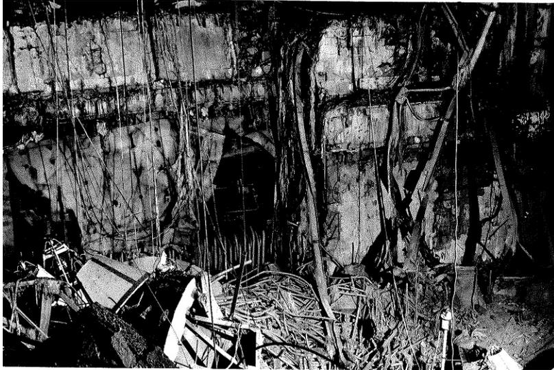
FIG. 36. Chernobyl NPP core damage. (Courtesy of Chernobyl NPP, Ukraine.)
