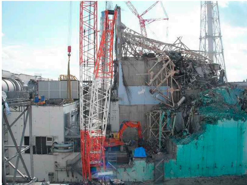
FIG. 22. Whole view of Unit 3 reactor building north side (before large debris removal). (Courtesy of TEPCO, Japan.)
