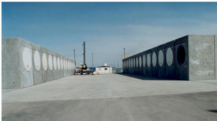
FIG. 49. Placement of TMI-2 fuel debris canisters into long term dry storage. (Courtesy of USDOE, USA.)
