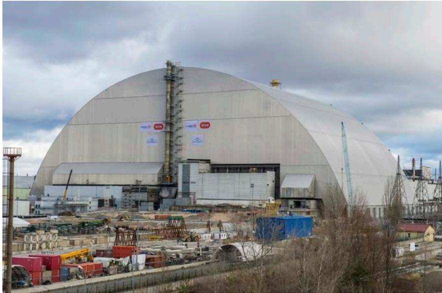
FIG. 1–3. NSC in the final position over the Unit 4. (Courtesy of Chernobyl NPP, Ukraine.)
