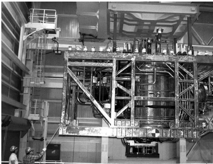
FIG. 54. Defence waste processing facility melter assembly prior to installation. (Courtesy of USDOE, USA.)
