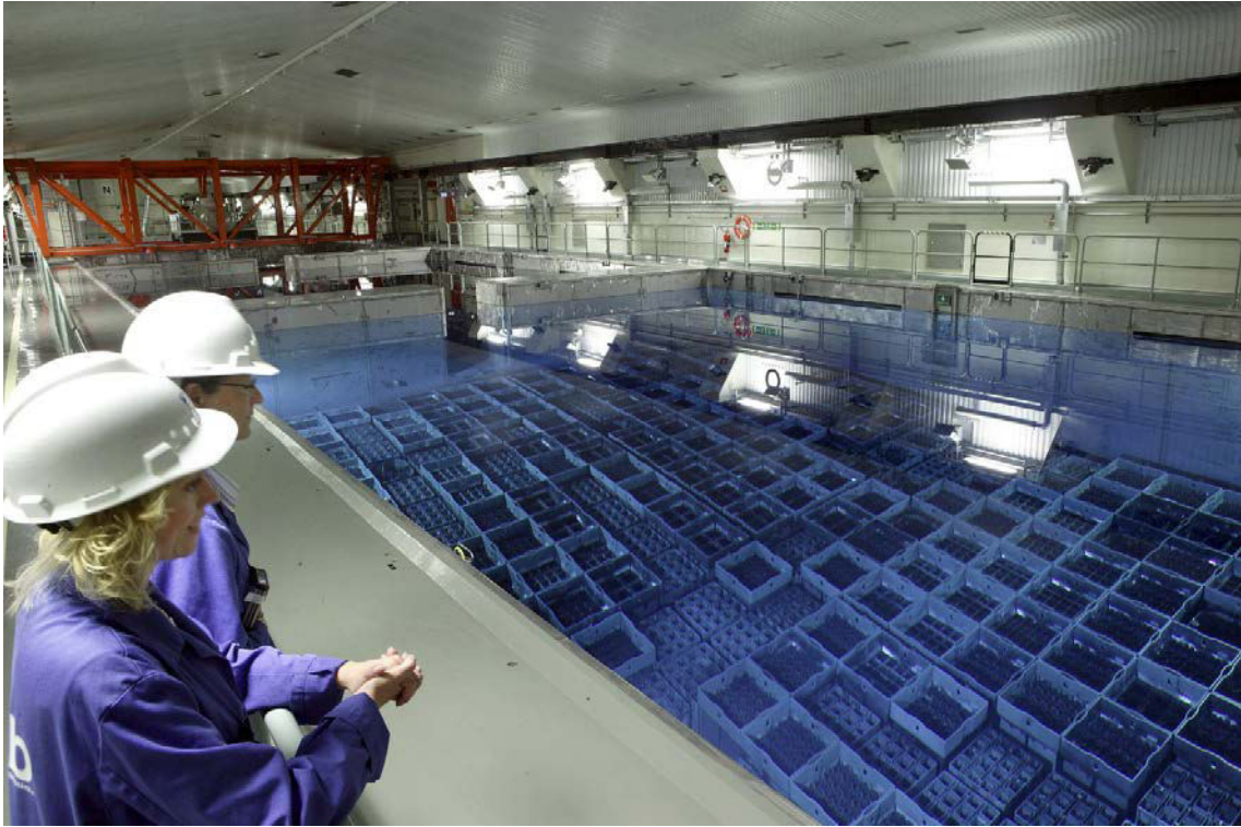
FIG. 7. The interim storage of spent fuel at Clab, Sweden (courtesy of SKB).
