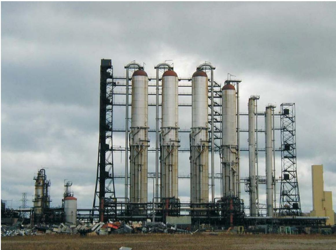
FIG. 25. Enrichment unit E4 of plant B (87 m high and 8.5 m in diameter) [109].
