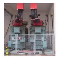
Fig. 7, Multisecondary transformers.
