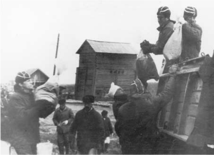
Photo 7. Removal of contaminated soil and snow from Georgievka.
