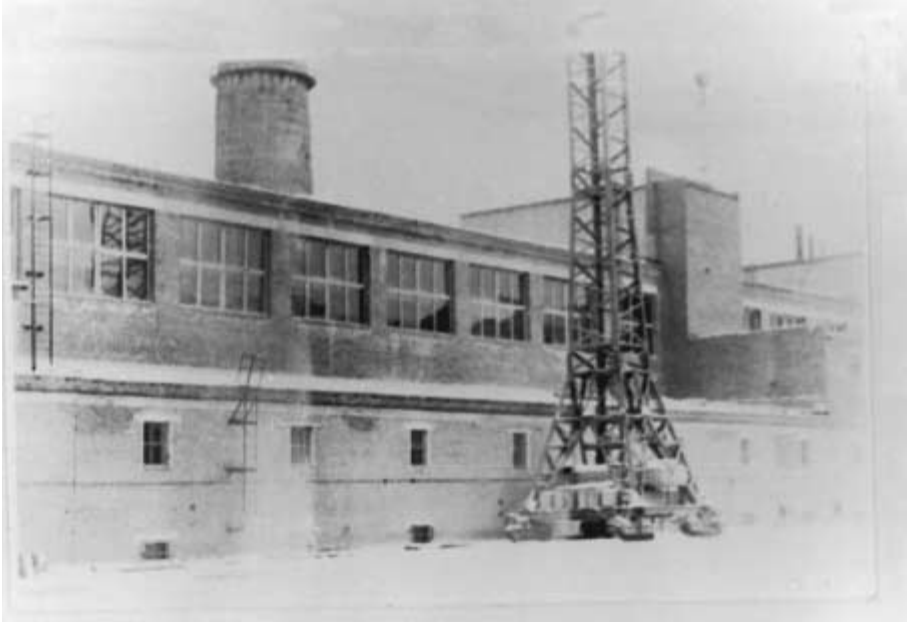
Photo 4. View of Building 201 after restoration.
