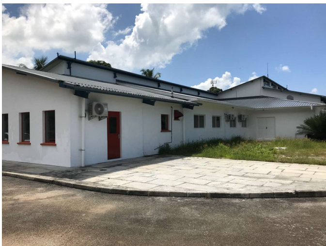
The wing of the new multipurpose laboratory where the Entomology Unit is located and that contains the infrastructure for future reception and handling of sterile flies.
