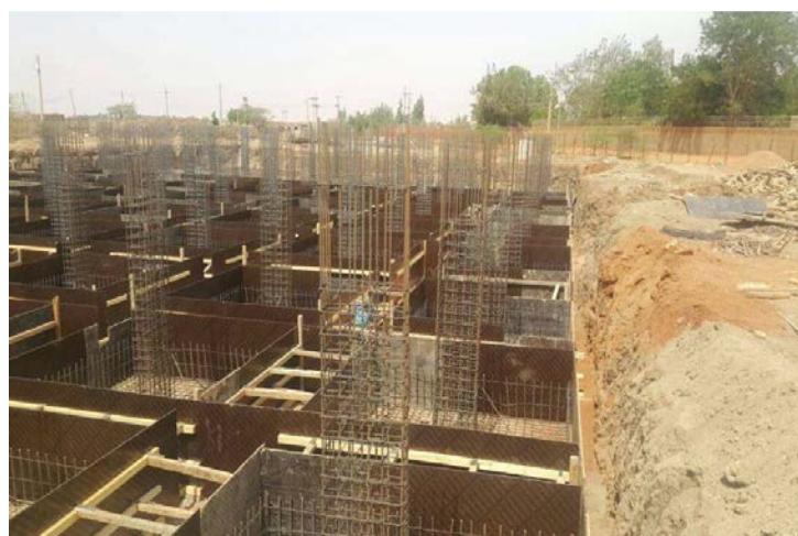
Construction of the Anopheles arabiensis mosquito mass-rearing facility in Soga, Khartoum, Sudan.
