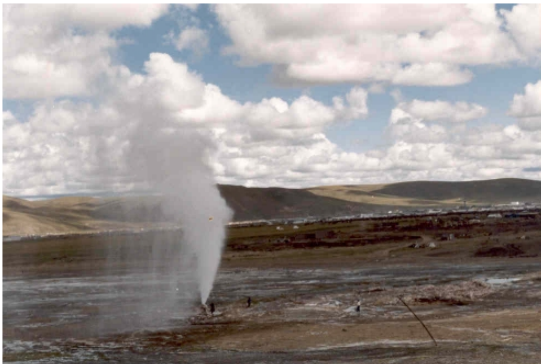
A geothermal well in vertical discharge in Naqu, Tibet
