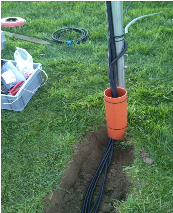
Installation of soil moisture cable network at the Grabenegg experimental station
