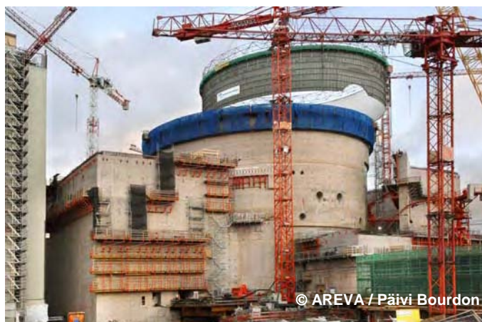
Construction of EPR at Olkiluoto - Finland
