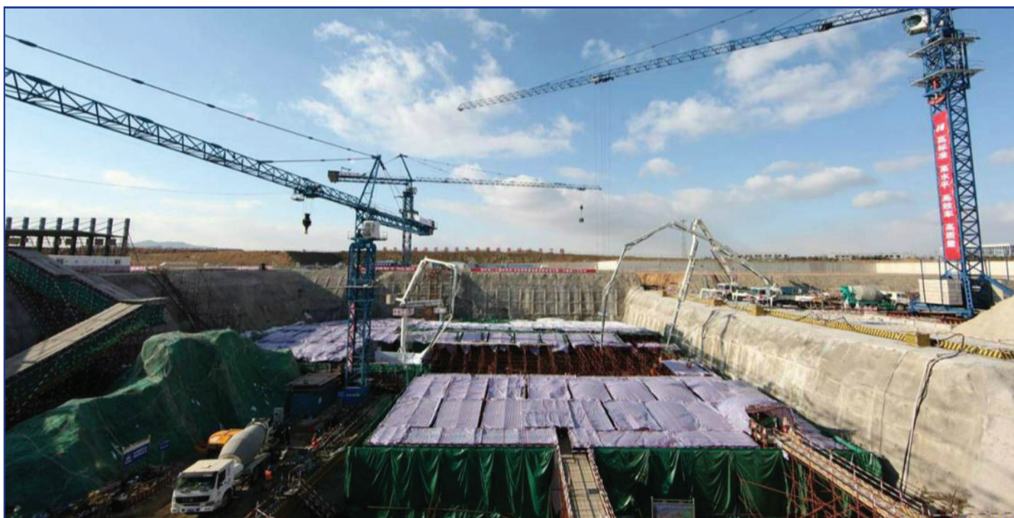
Currently under construction in east China's Shandong Province: the High Temperature Reactor – Pebble-bed Module (HTR-PM).
