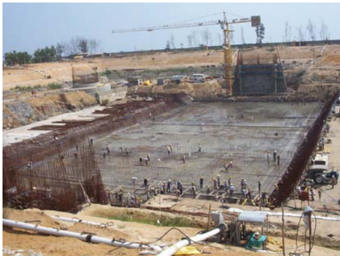
PFBR Construction Site, Kalpakkam, India (Credit: IGCAR)
