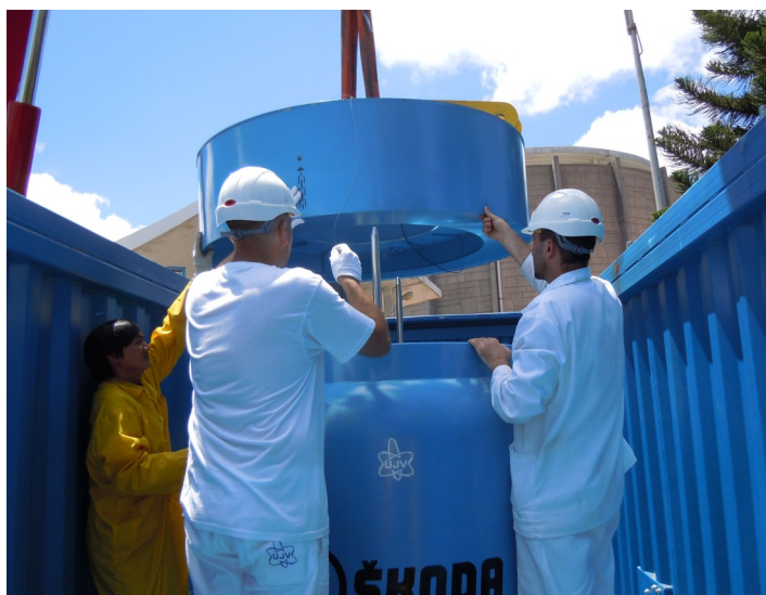
Fitting the upper shock absorber on top of the VPVR/M container.
