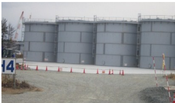
Temporary storage of contaminated water in above ground tanks and underground reservoirs. (Photos: TEPCO)
