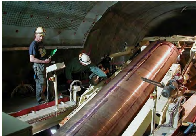
Testing technologies for SNF disposal: deposition of canisters (Äspö Laboratory, Sweden)
