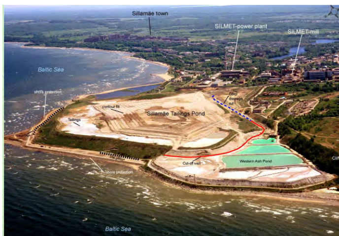
Fig 1. Remediation of the Sillamäe Radioactive Tailings Pond in Estonia.
