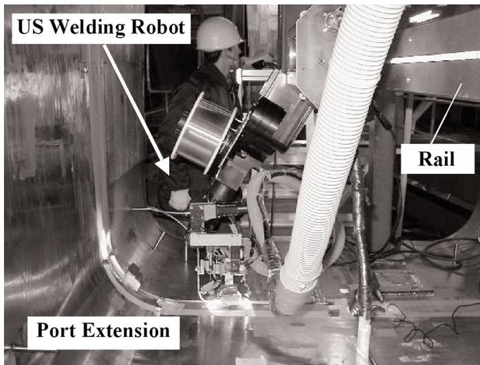
Fig. 4. Port extension assembled to VV sector (JAPT, USPT, RFPT)
