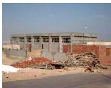
Figure 1: Main Building of Test Facility
