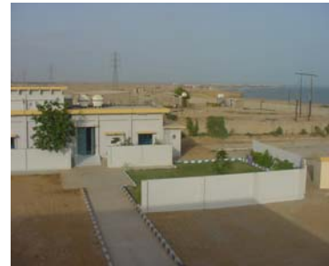
SWRO Plant at KANUPP
