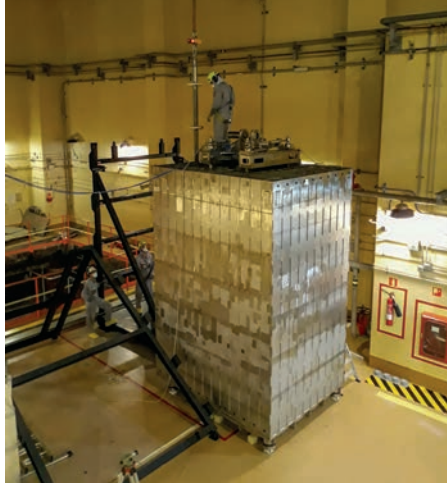
FIG. 9. Pressurized water reactor (PWR) storage rack. Courtesy ANAV (Asociación Nuclear Ascó – Vandellós II).
