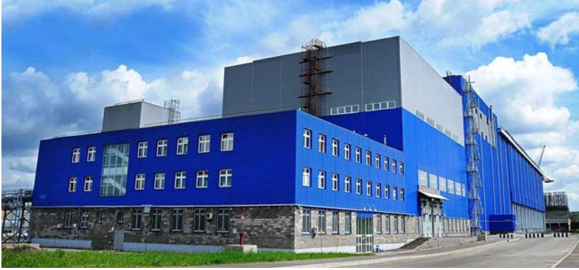
FIG. 58. General exterior view of the dry RBMK spent fuel storage facility.
