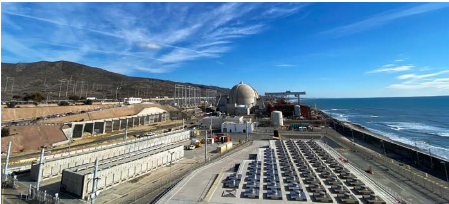
FIG. 67. SONGS TN NUHOMS (left) and Holtec UMAX (right) Storage Systems. (Courtesy of SCE.)
