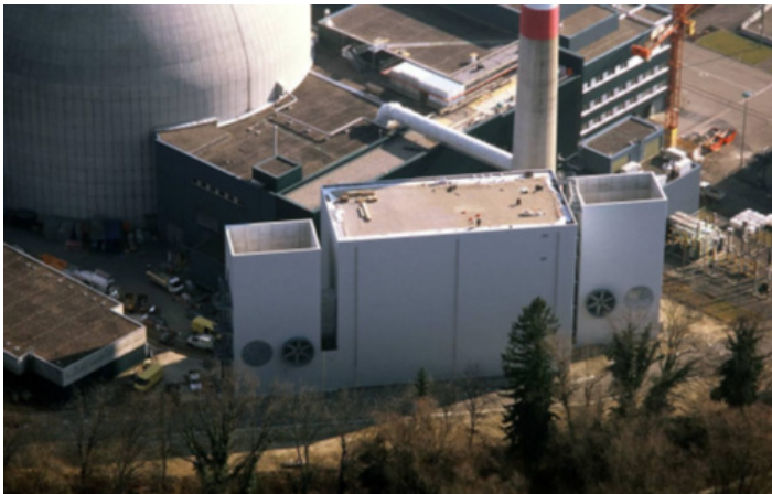
FIG. 64. Completed wet storage facility at KKG, Switzerland.
