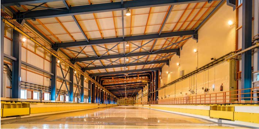
FIG. 40. Storage hall of MVDS at Paks NPP Hungary.
