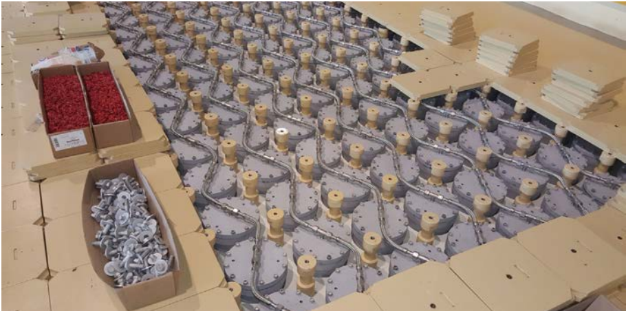
FIG. 41. Detailed view of the top of the storage tubes at Paks NPP Hungary.
