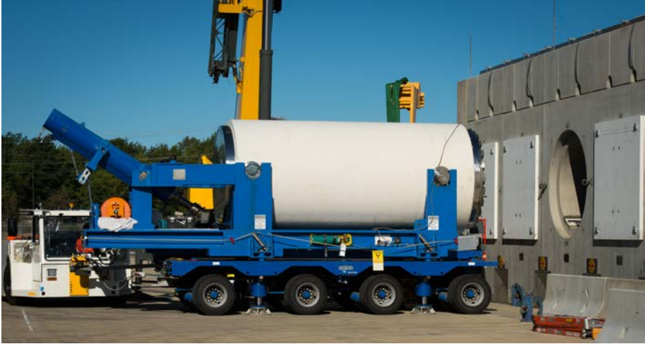
FIG. 37. Loading the canister into a horizontal concrete module (Orano's NUclear HOrizontal Modular Storage system known as NUHOMS, TN Americas).
