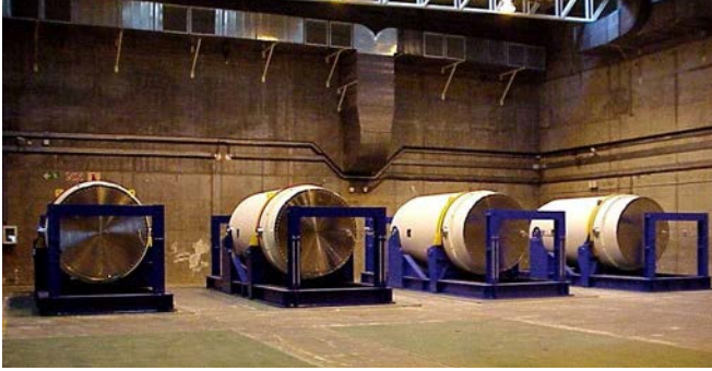
FIG. 19. Horizontal storage at Koeberg, South Africa (courtesy of Gesellschaft für Nuklear-Service).
