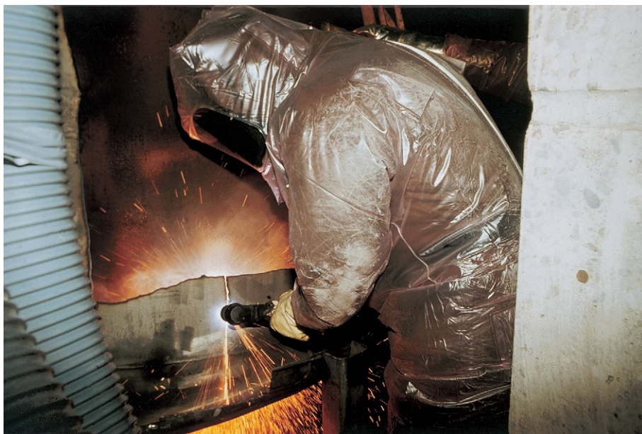
FIG. 29. Plasma cutting of metal components.
