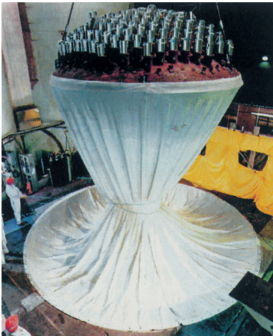
FIG. 52. Removal of the WAGR top dome.
