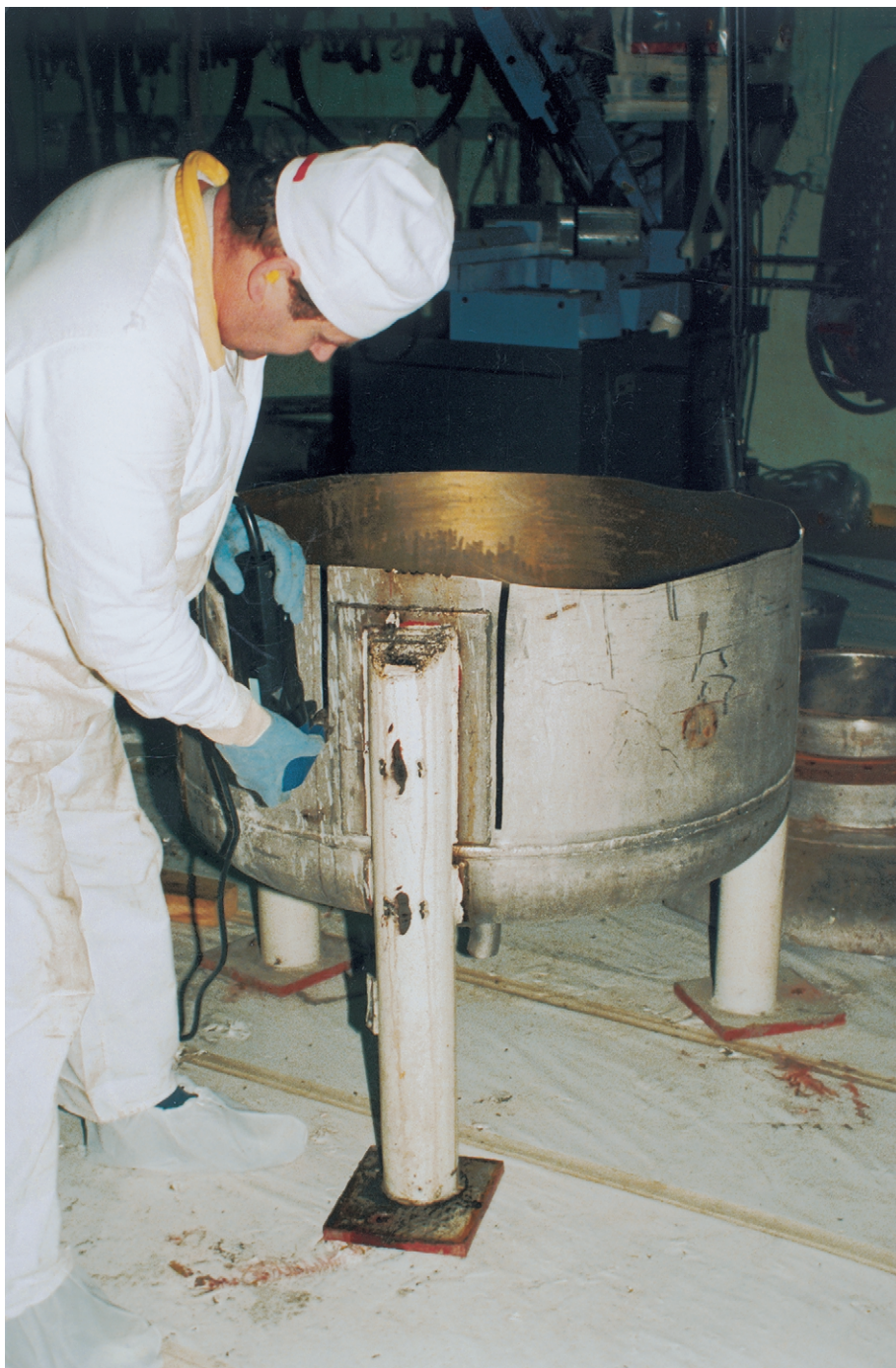
FIG. 16. Nibbler cutting thin plates, BR3 decommissioning project.
