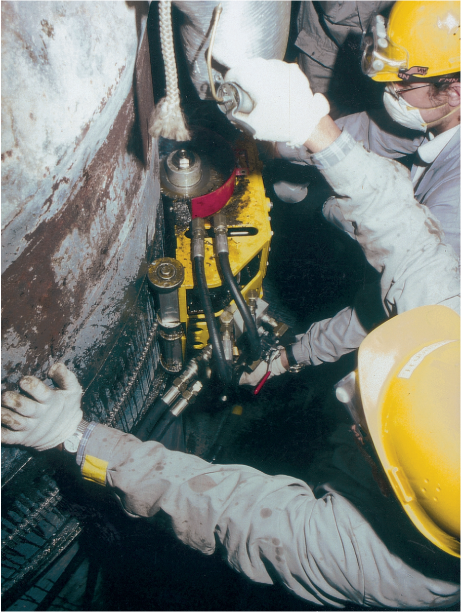
FIG. 21. Circular cutter in use at the HDR facility in Germany.
