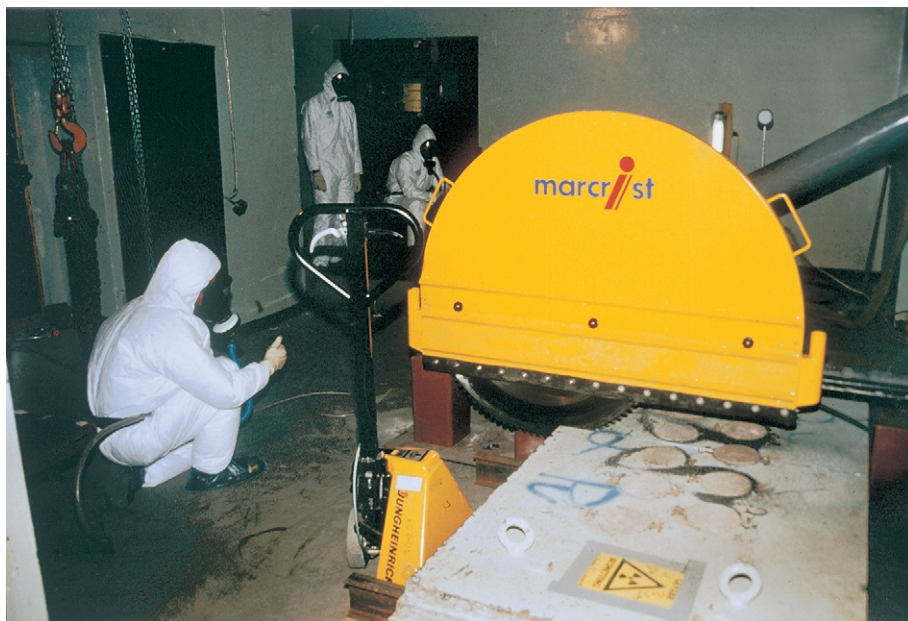
FIG. 22. Dry cutting of cast iron shielding blocks using diamond tipped blade saw.
