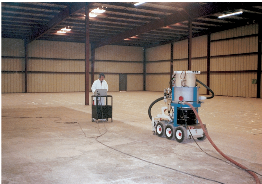
FIG. 49. Scabbling robot at work.
