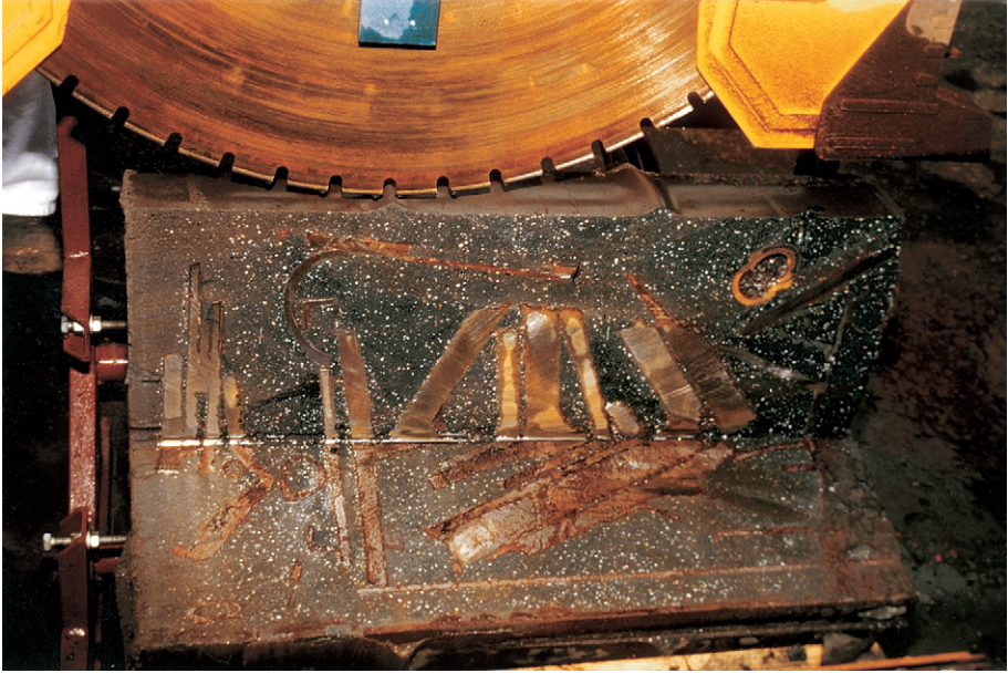
FIG. 24. Concrete cutting using a diamond tipped blade saw.
