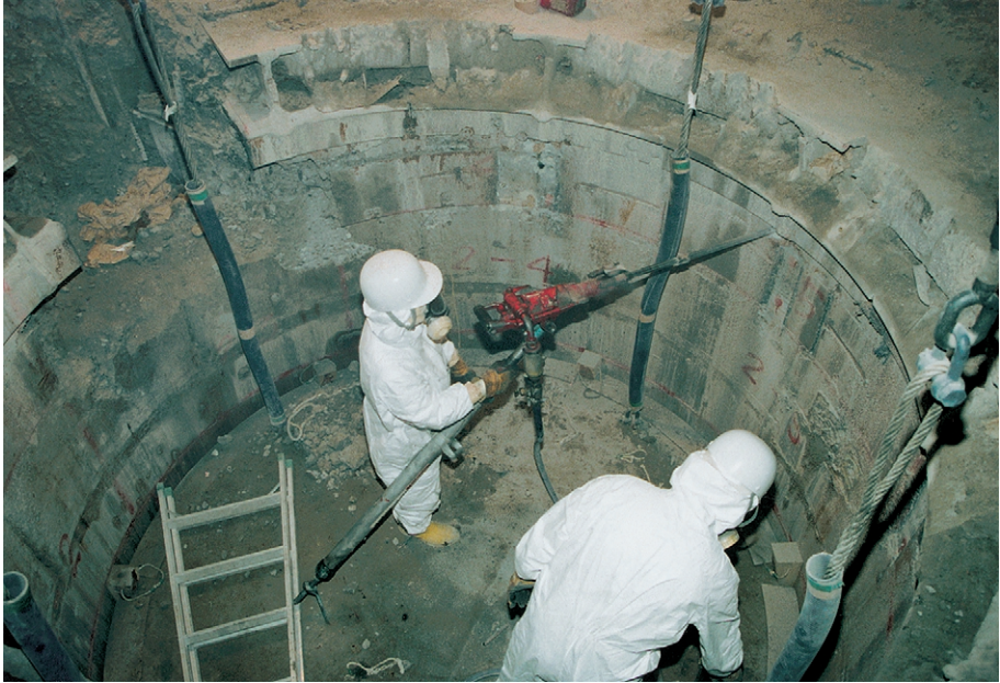
FIG. 26. Drilling being carried out for the insertion of explosives prior to the demolition of biological shield structures by controlled blasting, JPDR decommissioning project.
