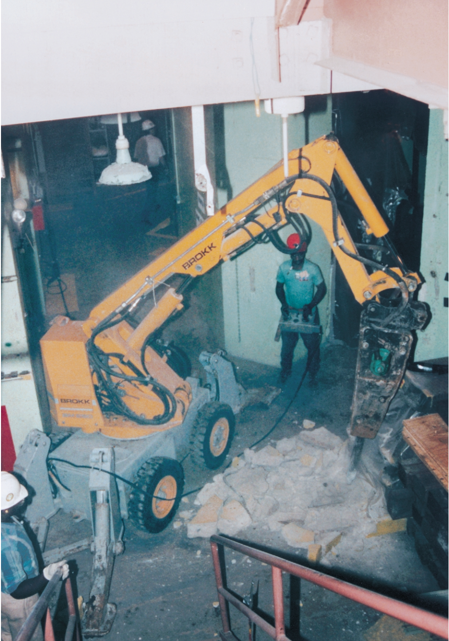
FIG. 40. Excavator being used for concrete removal at EBWR. Courtesy Argonne National Laboratory, managed and operated by the University of Chicago for the US Department of Energy under contract No. W-31-109-ENG-38.
