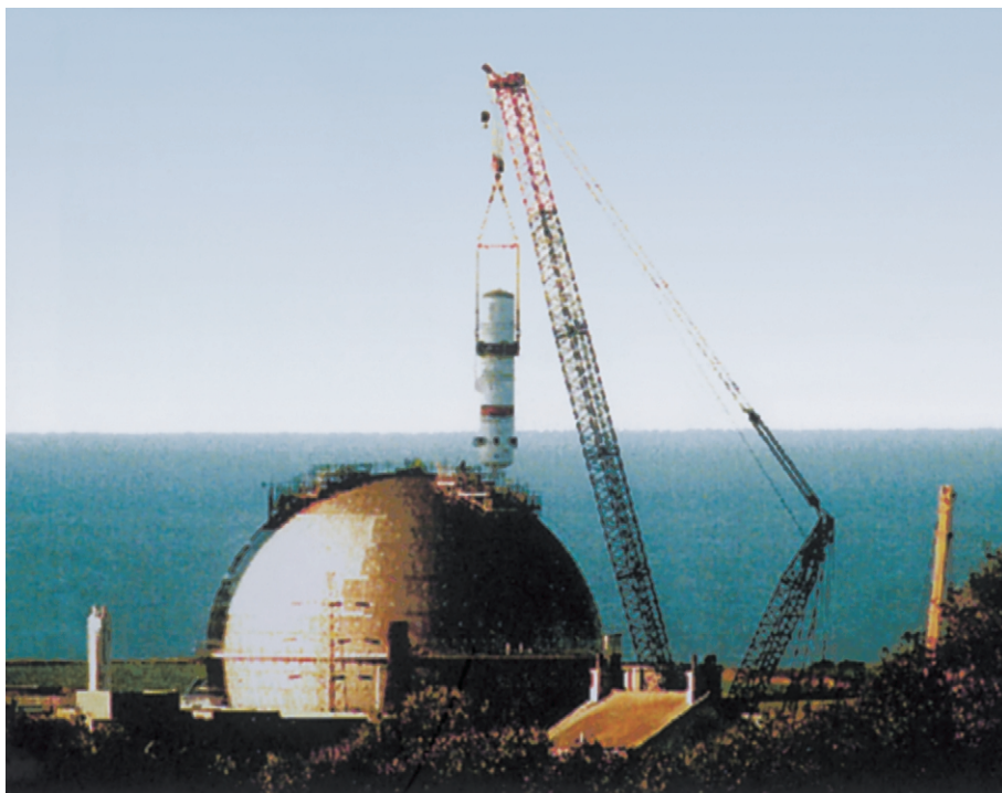
FIG. 54. A heat exchanger being removed from the WAGR.
