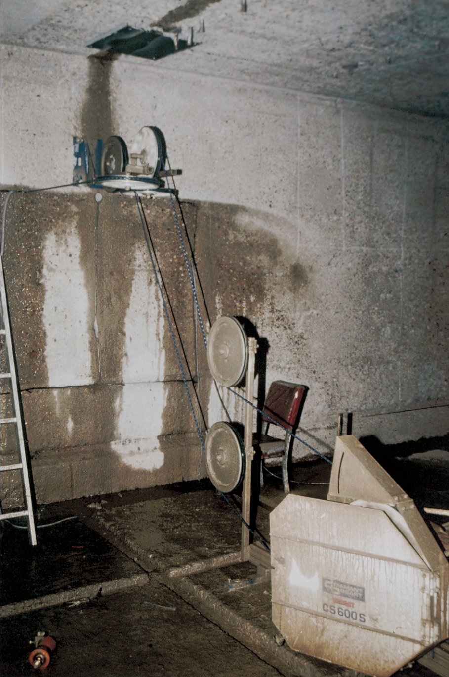
FIG. 23. Creating new cell entrances using a diamond cable cutting machine.
