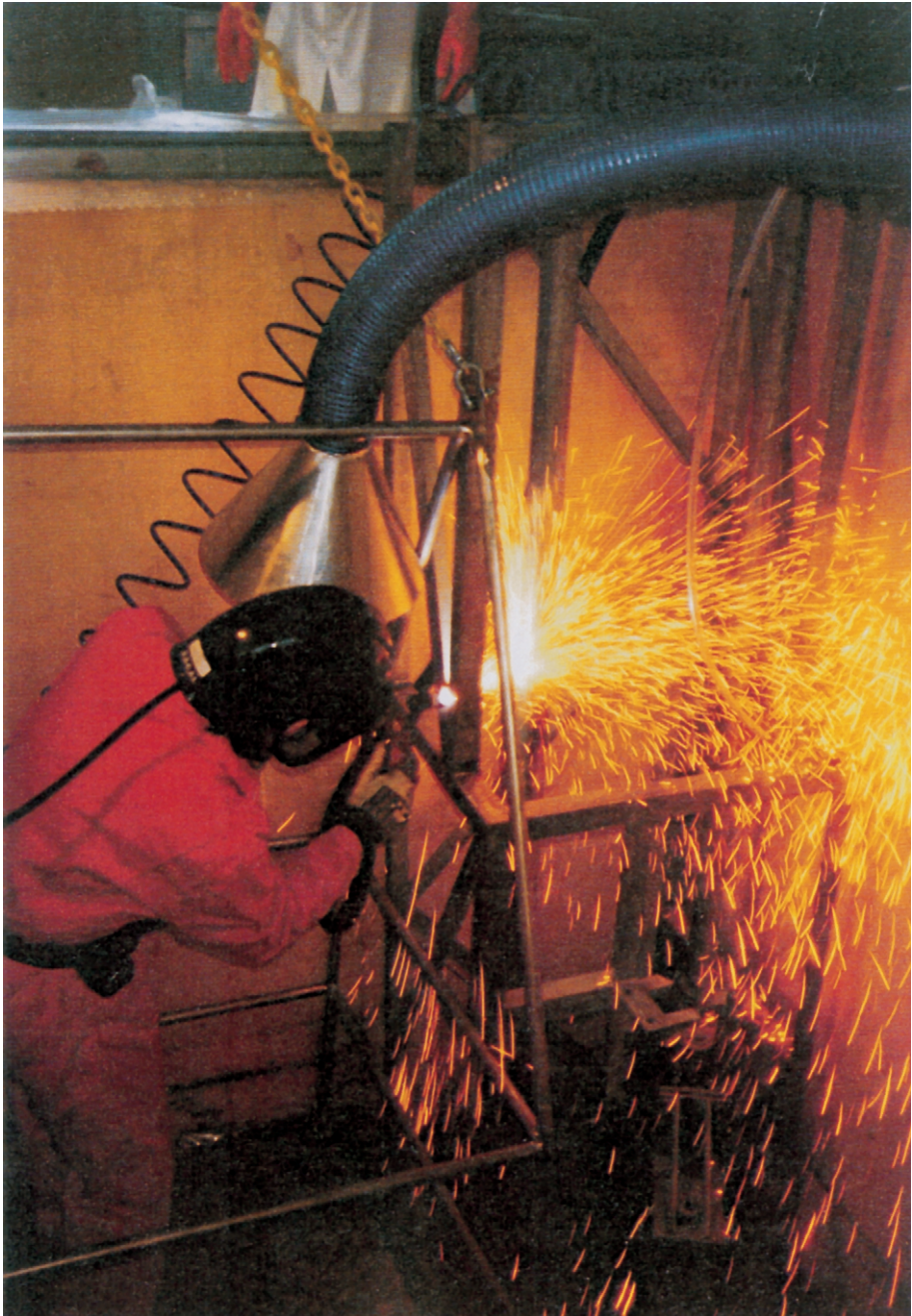
FIG. 30. Plasma arc cutting being used during the removal of the equipment employed for decanning uranium elements, Kjeller reprocessing plant, Norway.
