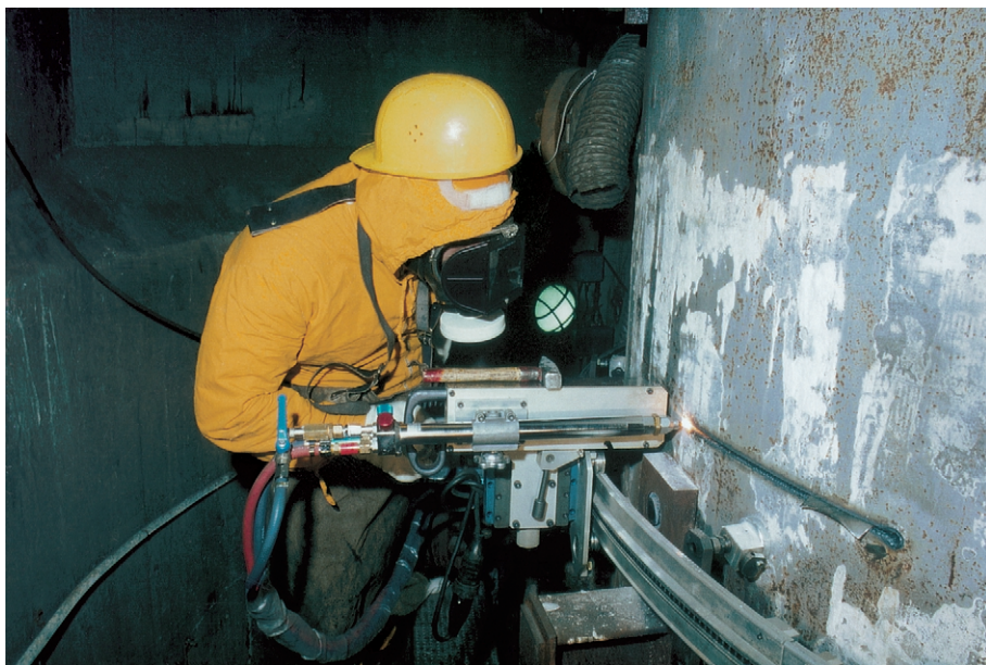
FIG. 33. Thermal cutting at HDR in Germany.
