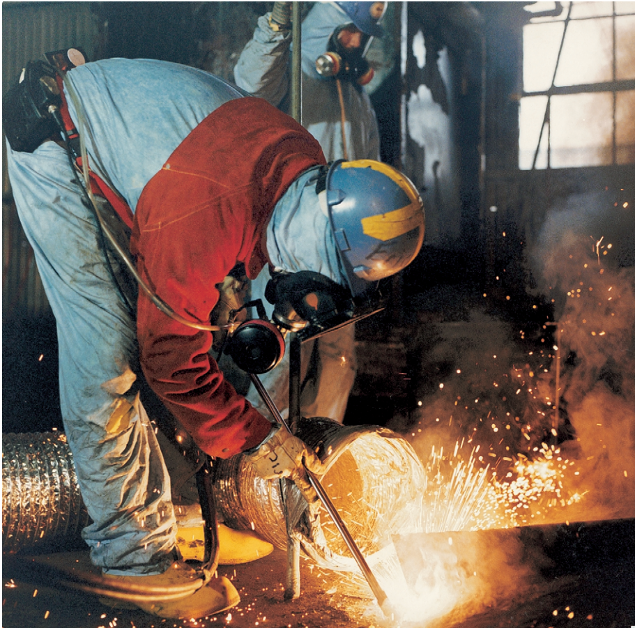
FIG. 32. Oxygas cutting equipment in use at the Fernald facility, USA.
