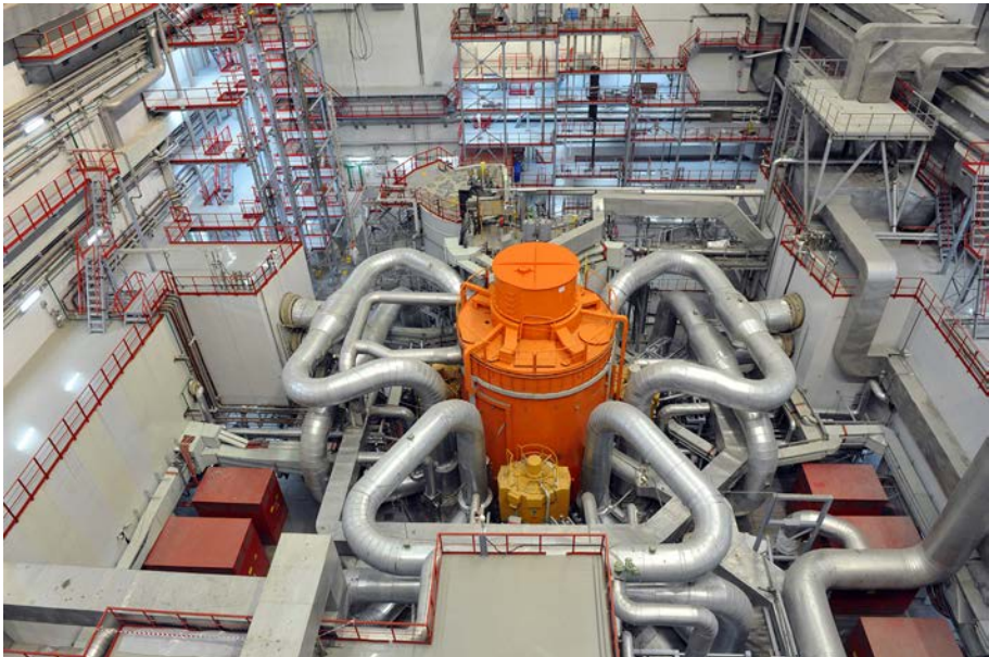
FIG. 27. Fast reactor BN-800 at the Beloyarsk nuclear power plant, Russian Federation. Reproduced courtesy of Rosenergoatom.
