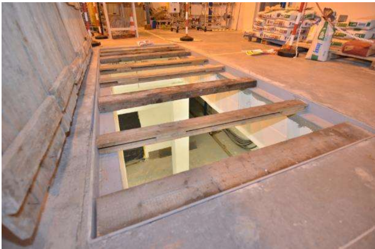
FIG. 9. Photo of rectangular floor opening for the cooling channel installation.
