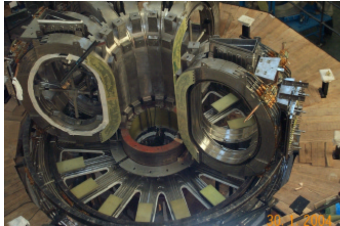
FIG. 5. TF modules on the support beams
