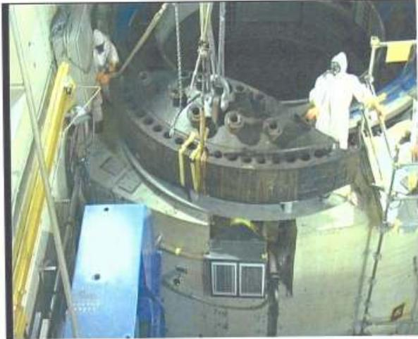
Fig. 13: First segment of RPV closure head onto its temporary position on the barge
