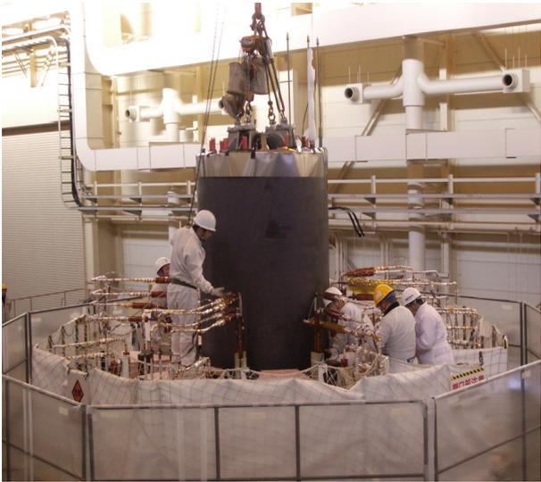
Fig.3 PFI coil installed in CSMC
