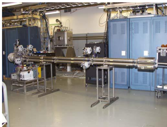
Fig. 4 The IPI gas removal system at ORNL
