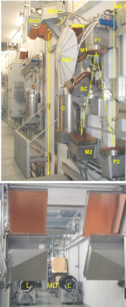
*FIG. 3. The W7-X quasi-optical transmission system. Top: Single beam section with BMO (M1, M2), short-pulse calorimeter (C), polarizers (P1, P2), microwave absorbers (AB1) and feeder mirror (M3) mounted on a common base frame. The beam path is indicated. Bottom: Section of the Multi-Beam-Waveguide, both cw-loads (L) are seen in the background.*
