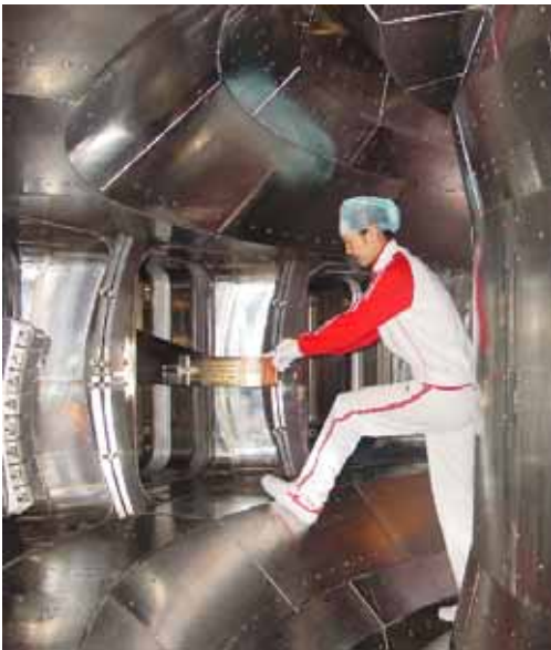
Fig.6 In vessel components installation
