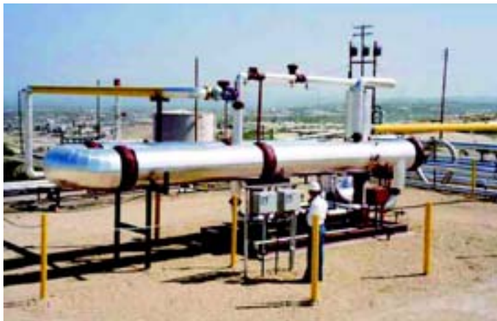
FIG. 3. Nucleonic gauge for oil, water and gas flow rate measurement during oil production in an oilfield.
