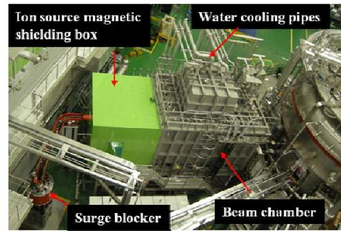
FIG.10. NBI-1 system in experimental hall
