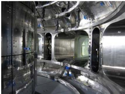
FIG. 7. IVCC segments installed in the vacuum vessel
