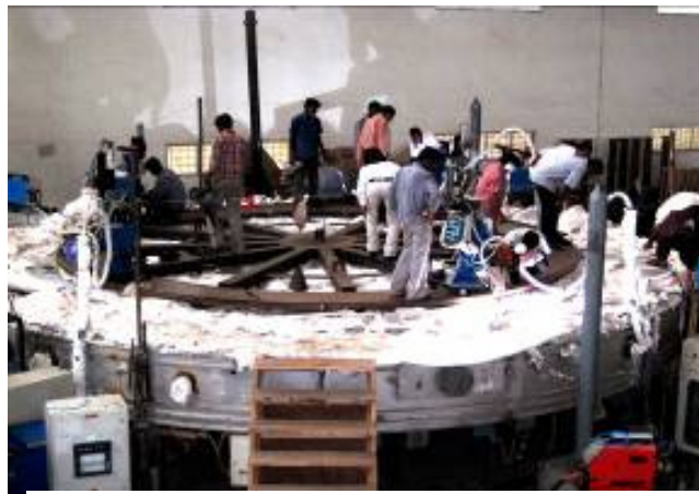
Hard Facing in Progress
