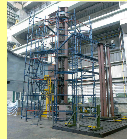
Transfer Arm Assembly in progress
