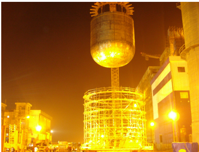
Erection of main on reactor vault in Dec '09
