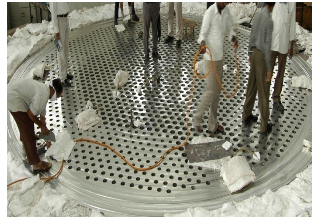
Preparatory work for hard facing
