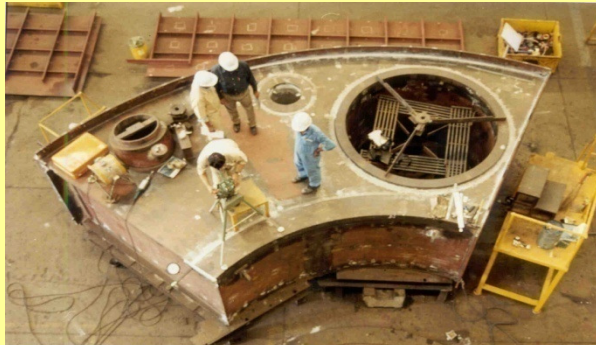
Sector of Roof Slab
