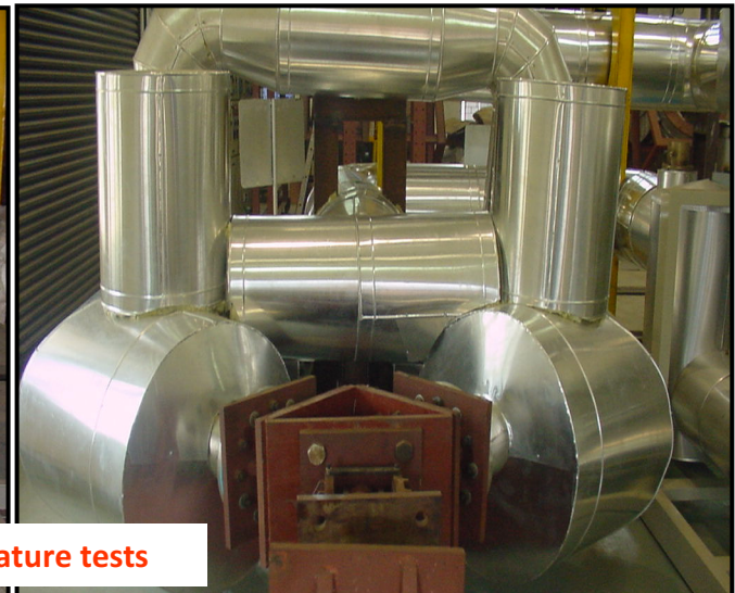
Pipe bends after insulation
