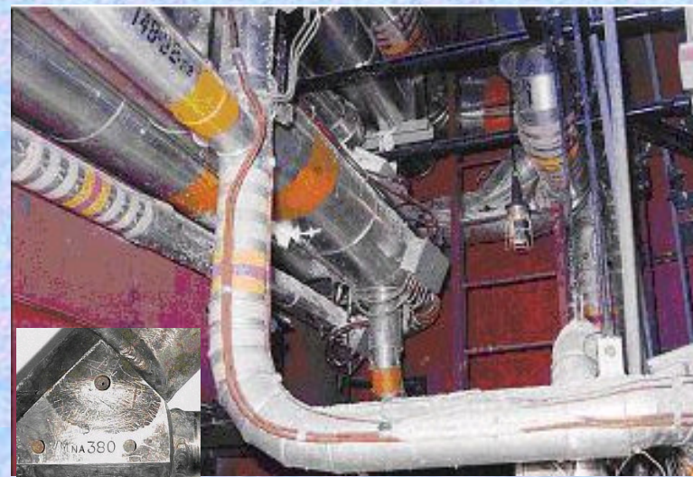
Sodium Leak inside Purification Cabin due to a hole in valve body
