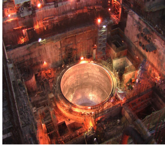
Erection of safety vessel on reactor vault in June'08
