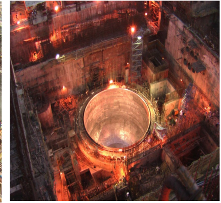
Erection of safety vessel in June 2009
