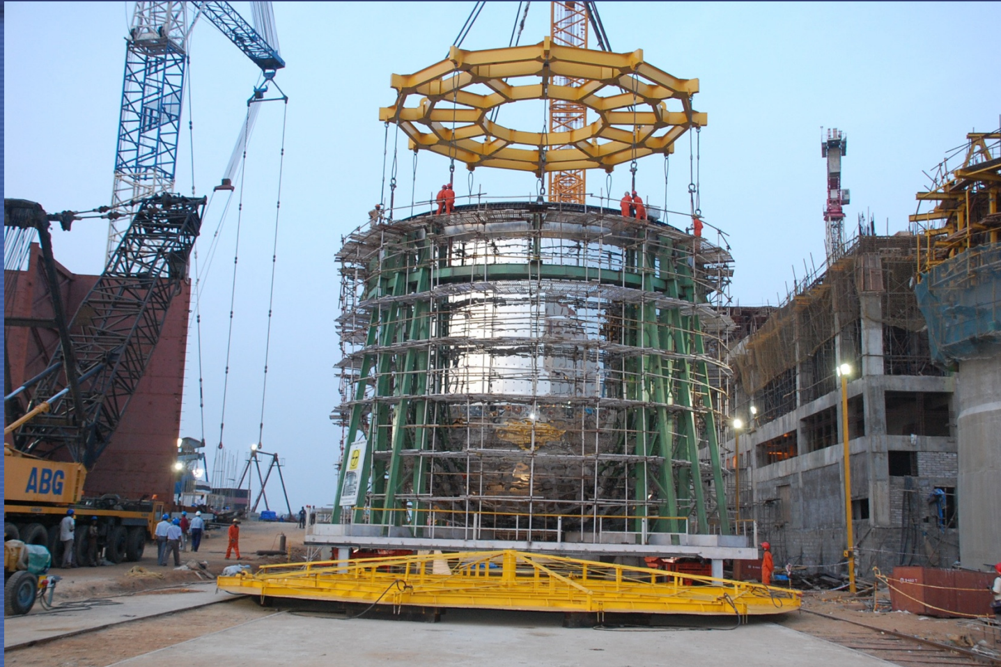
Safety Vessel ( \varnothing 13.5 m, H 13.5 m, 160 t) Transported from On-site Shop to Reactor Building (June 2008)
