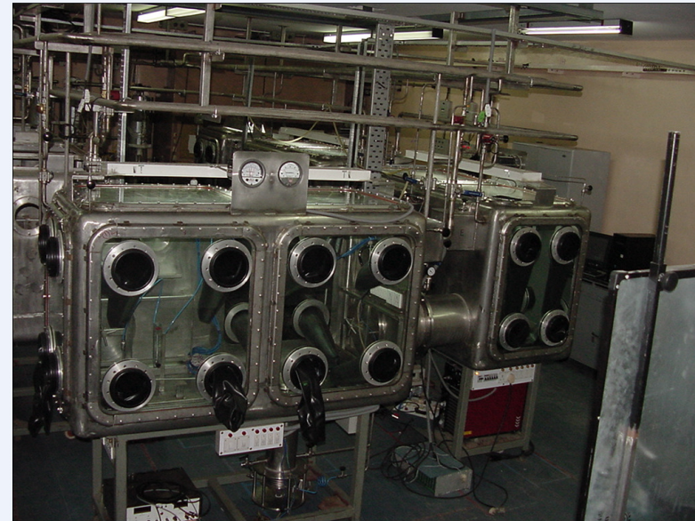
Sodium bonded pin fabrication facility
