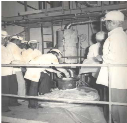
Charging of Sodium Bricks in Melter Tank
