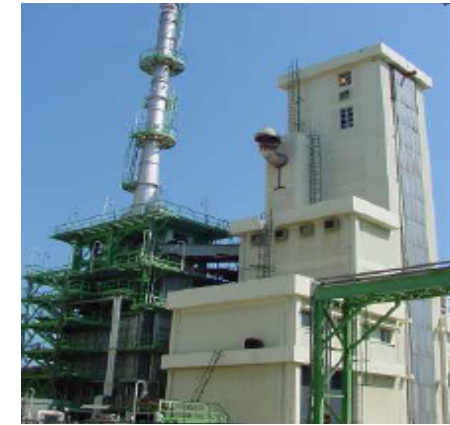
5.5 MWt Steam Generator Test Facility
