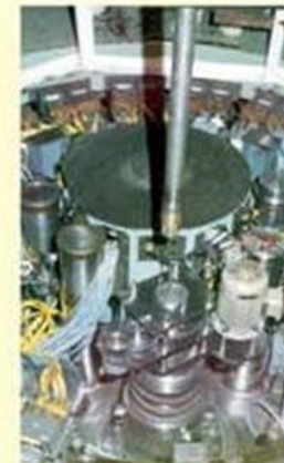
Guide Tube Cutting Machine Being Installed
