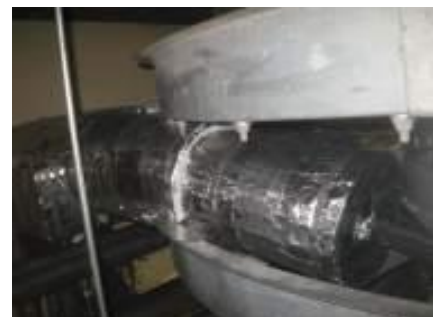
Cable Wrapping (7 layers)
